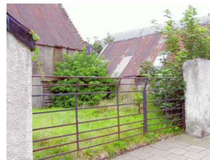
Left: Townlands Barn from High Street Right: Townlands Barn south elevation
