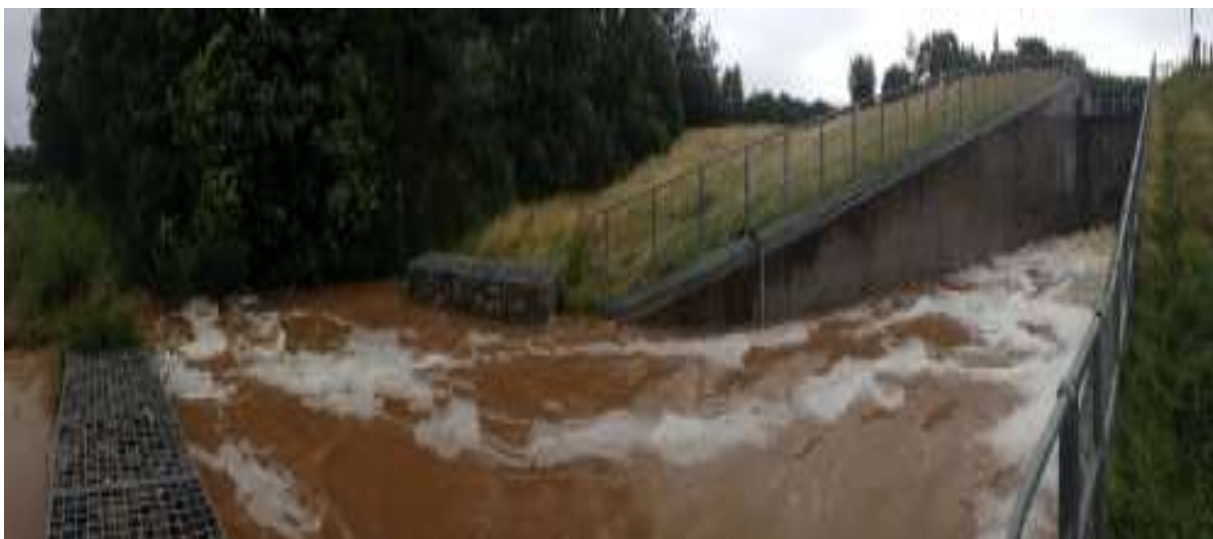
Lhanbryde Control Structure during flood event
