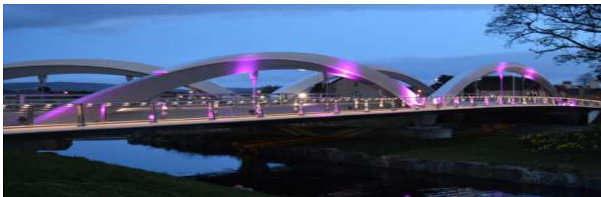
Elgin Flood Alleviation Scheme – Landshut Bridge
