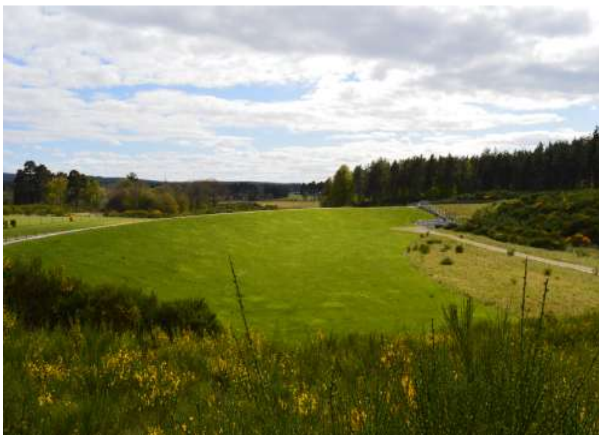
Chapelton Flood Storage Reservoir, Forres
