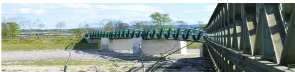
Broom of Moy Footbridge, Forres
