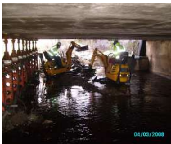
Burn of Rothes – Sediment Removal
