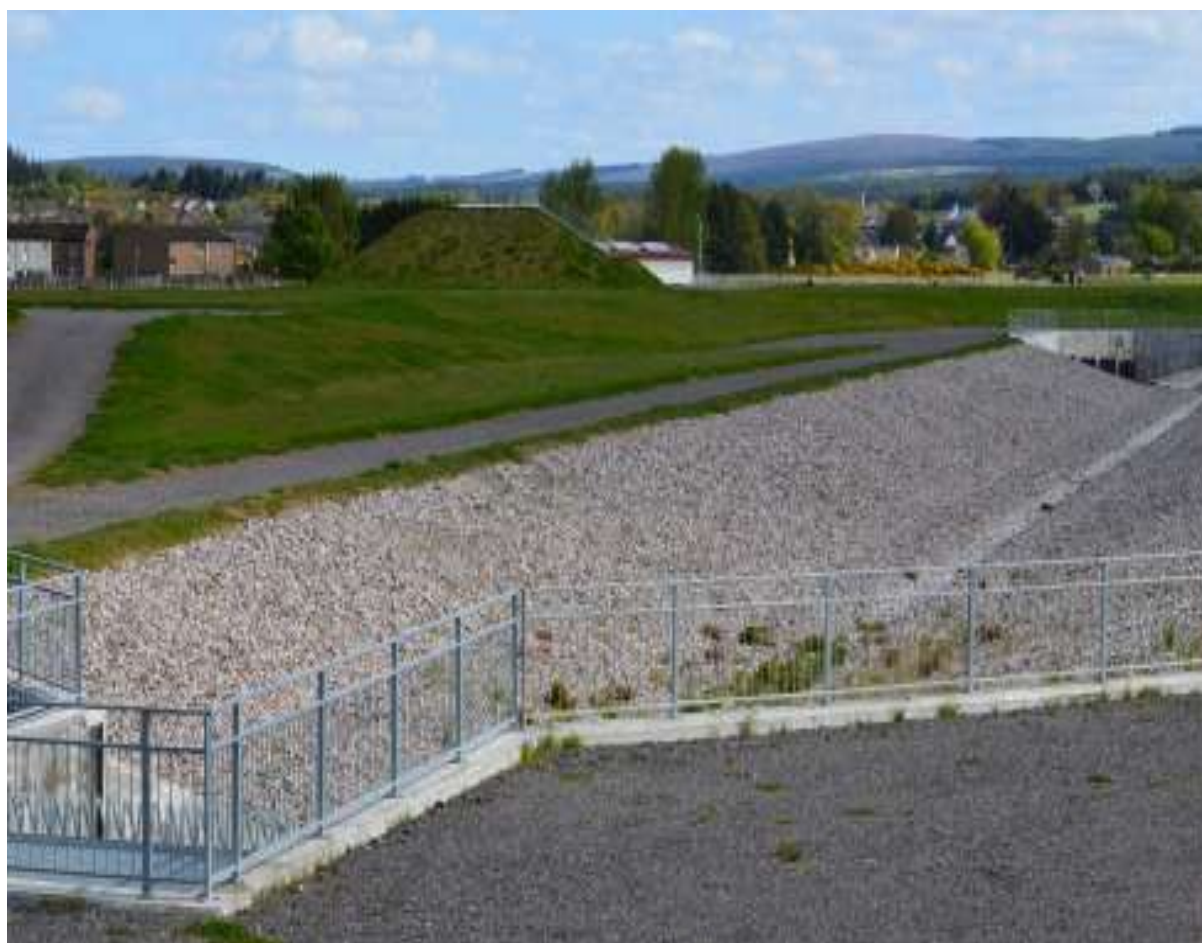
Pilmuir Drainage & Pumping Station, Forres
