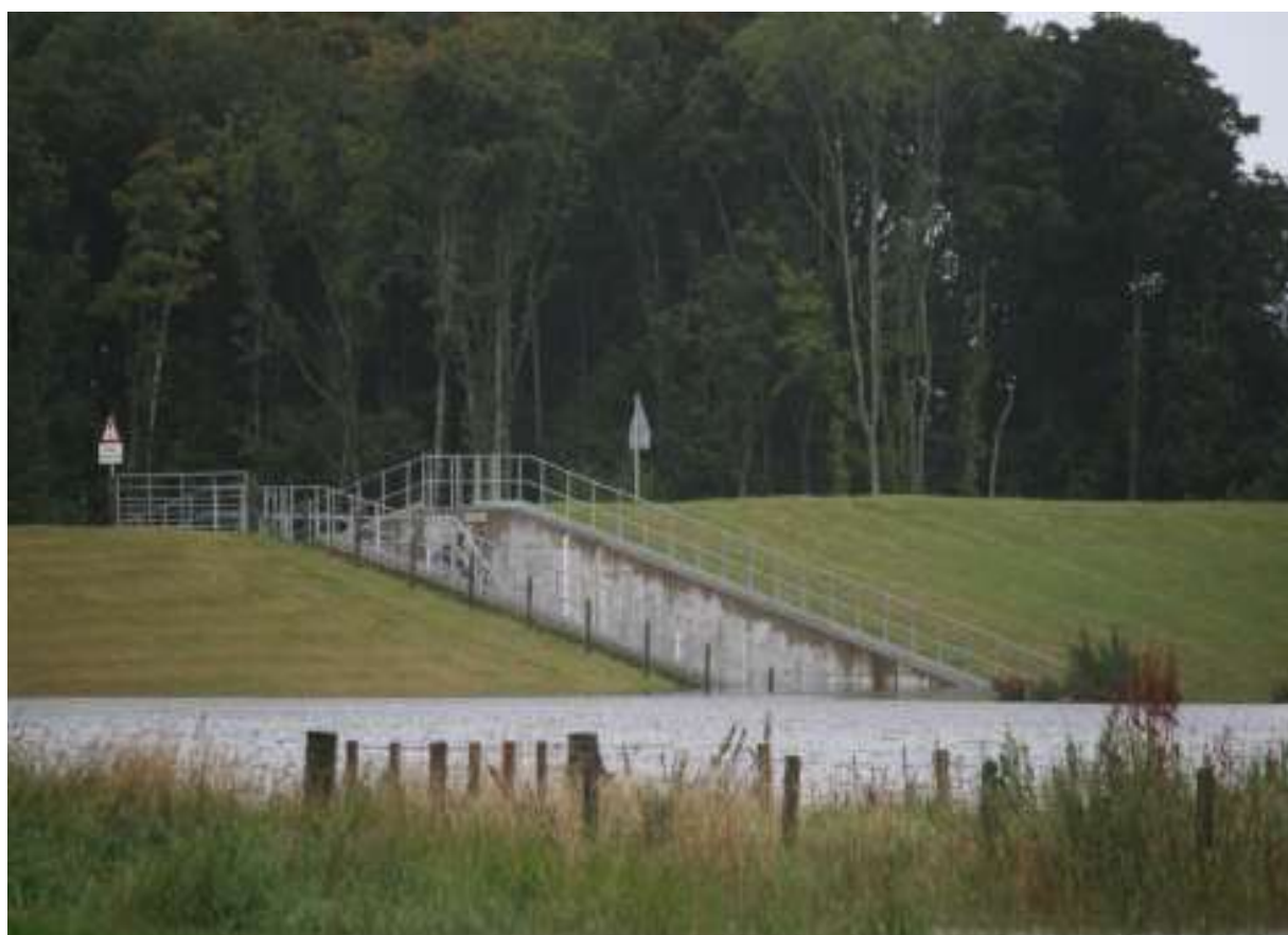
Lhanbryde Flood Storage Reservoir in operation
