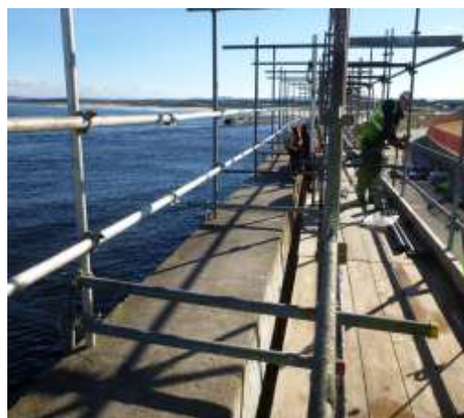
Lossiemouth Sea Wall Repairs
