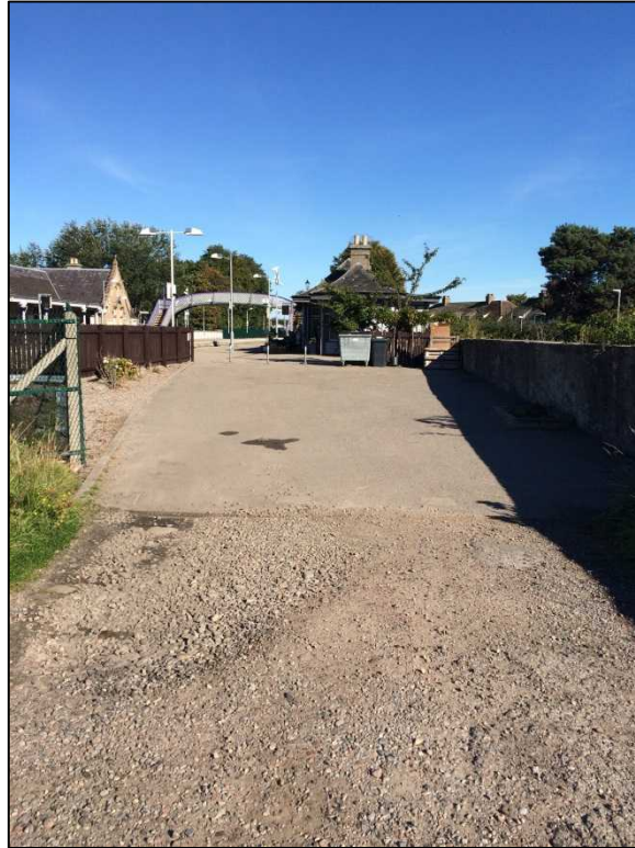
Photo BC3 – South platform ramp looking from secondary car park
