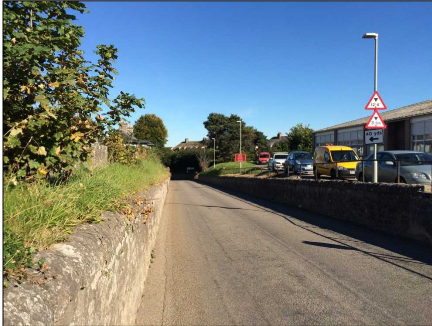
Photo BC1 – Balblair Road looking northeast towards the junction
