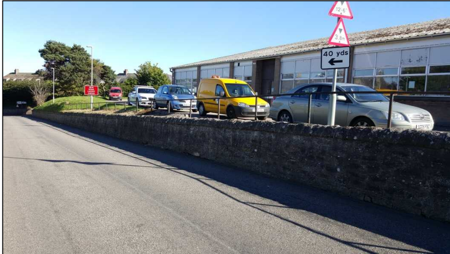
Photo BC4 – Balblair Depot retaining wall
