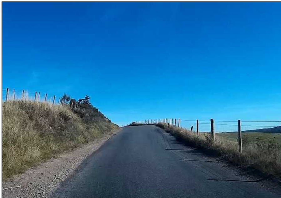
Photo D8 – Balblair Road facing north at entry to bend with carriageway widened on the inside of left-bend ahead (a gravel run-over area can be seen on left verge)
