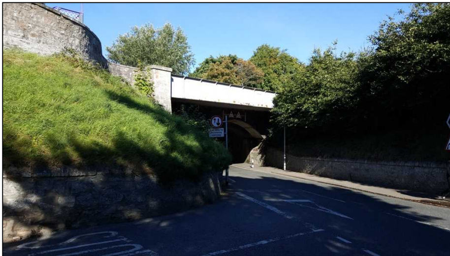
Photo BC5 – Balblair Road sightlines, southwest corner looking north towards bridge
