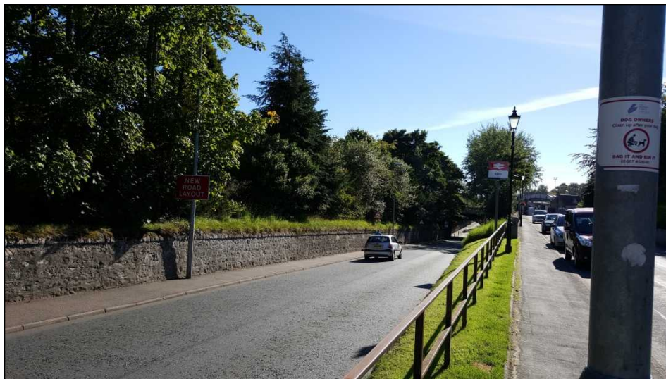
Photo C1 – Cawdor Road looking south towards bridge from Cawdor Street
