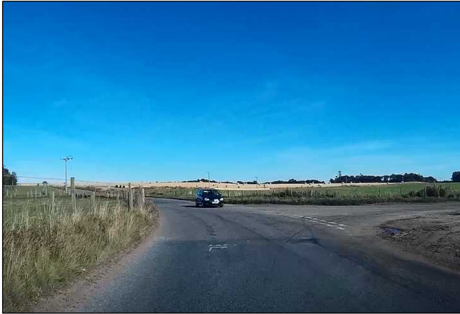
Photo D3 – Balblair Road facing north at junction of existing unclassified road linking to Cawdor Road to the south of the development area
