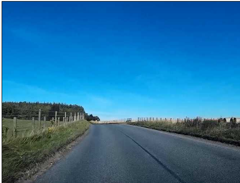
Photo D2 - Balblair Road looking north towards southern boundary of the Nairn South development area (located beyond field access seen on right)
