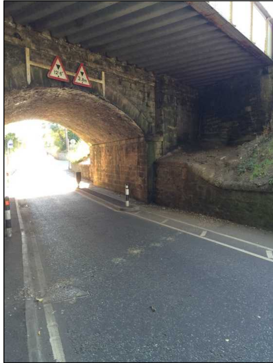
Photo C4 – Cawdor Road looking south through bridge arch
