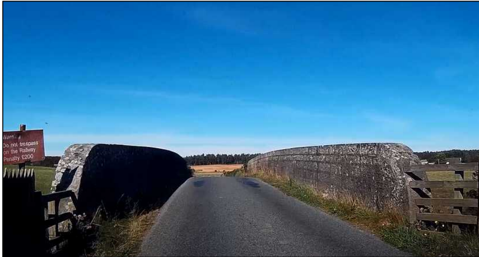
Photo D13 – C1163 Delnies Road railway bridge crossing
