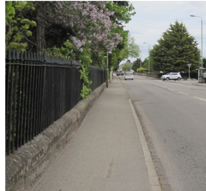
Simple, appropriate, easily repaired paving.
