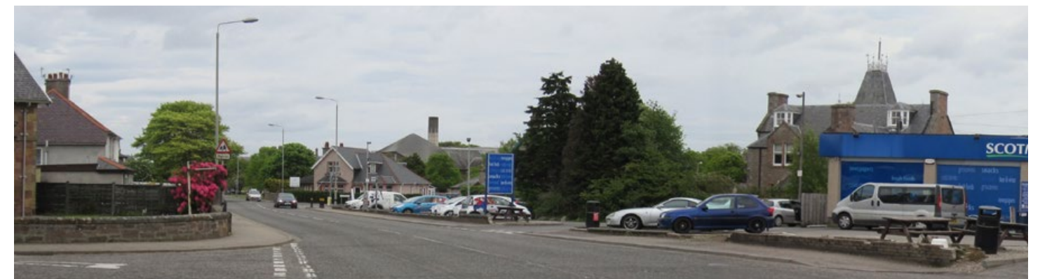
Open frontage and inappropriate building line detract from the character of the townscape.
