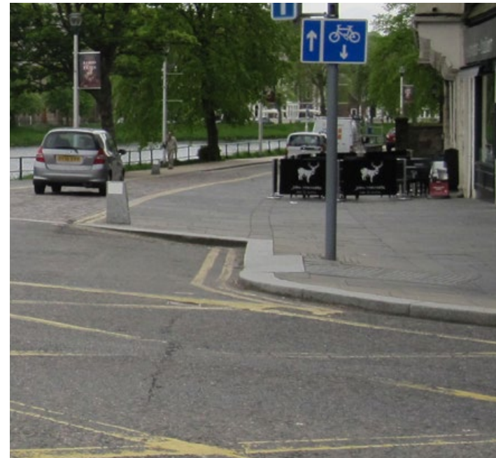
'Fat' kerbs: traditionally used for 'high streets' and important civic places. A distinction misunderstood by many designers and used in any 'improvement scheme'.
