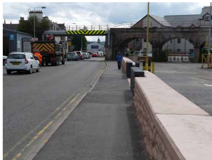
Widening the footway by about 1 m would create a safe shared surface
