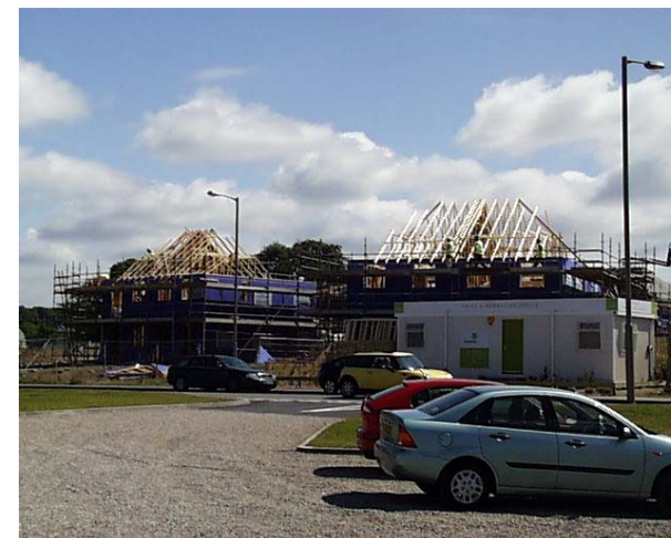
house-building at Inshes
