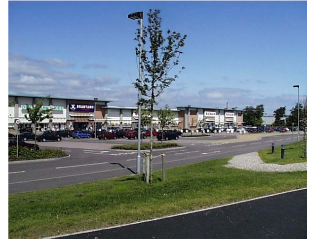
district facilities at Inshes
