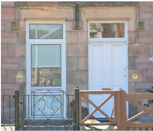
A half glazed inappropriate modern aluminium door, the poor finish, appearance and style accentuated by the adjacent traditional timber 4 panel double margin door.
