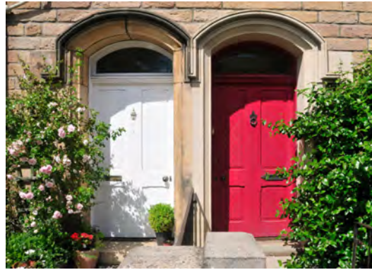
Pair of 4-panel doors with decorated panels and detailed moulding.
