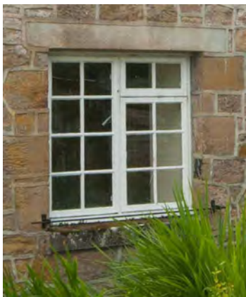
Multi-pane casement windows.
