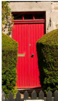
Double-leaf plank and batten door with top light.
