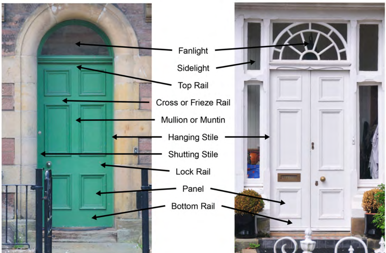
Figure 3.1 The anatomy of a traditional sash and case window and traditional doors.
