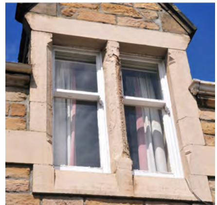
Note how the top sash projects over the lower sash. This example has 'horns'.
