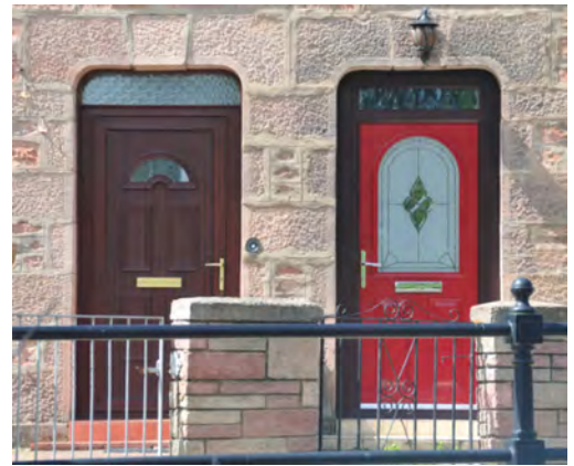
This pair of off-the-shelf uPVC and half glazed doors do not match one another as intended and also detract from the character of the building and wider area.
