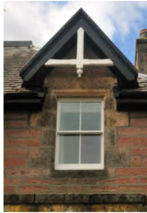
4-pane sash window.
