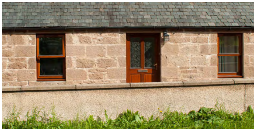
Timber effect uPVC door with glazed panels which detracts from the character and appearance of the traditional cottage.
