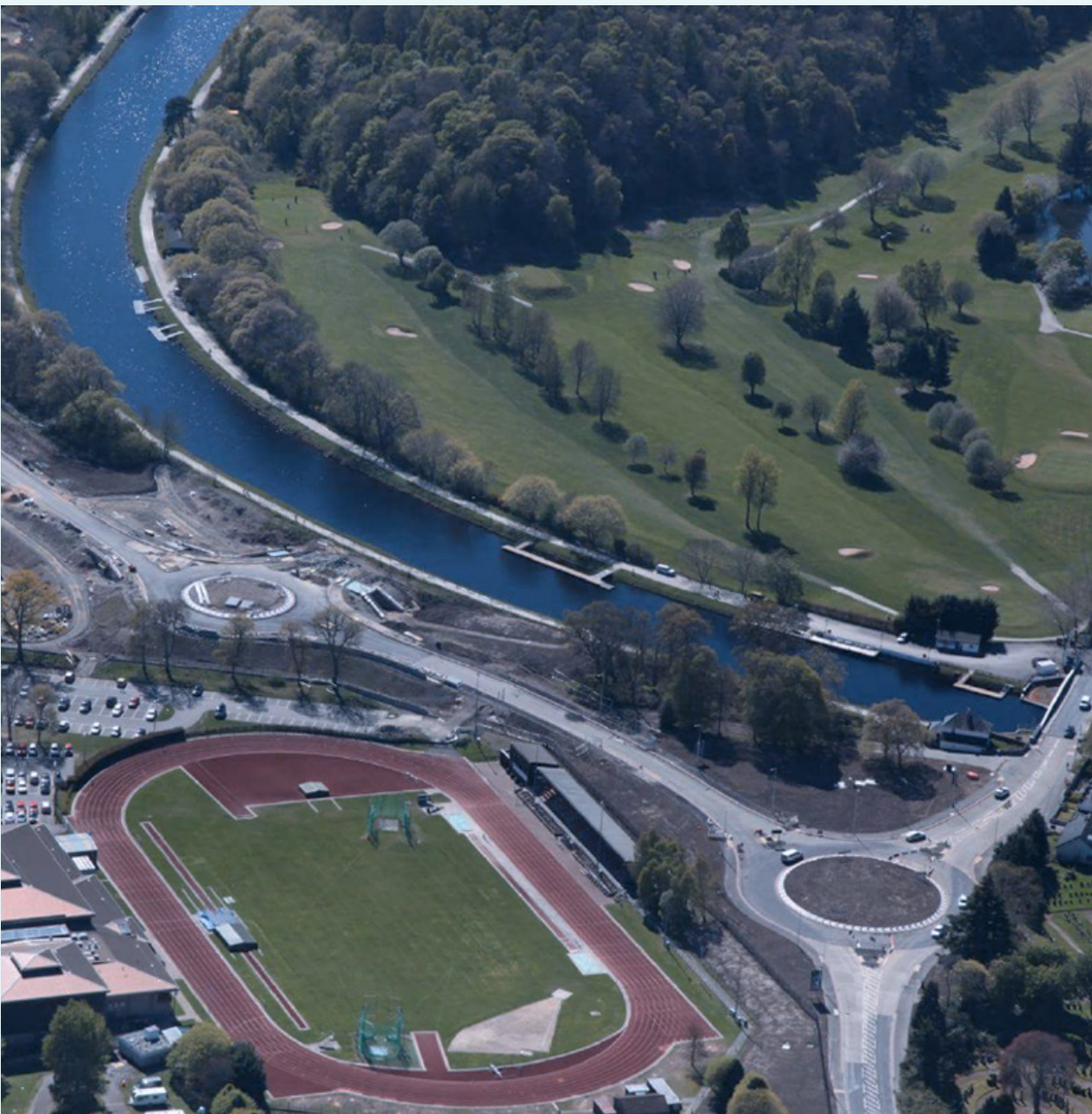
Phase 1 of the West Link Road Scheme is well underway.
