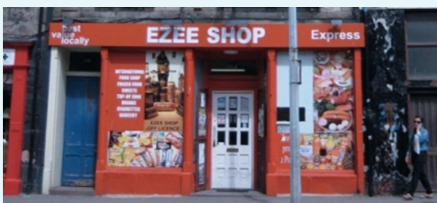
114 Academy Street - before improvement.
