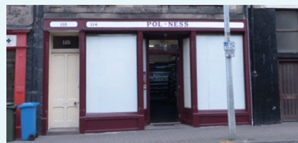
114 Academy Street - following improvement.
