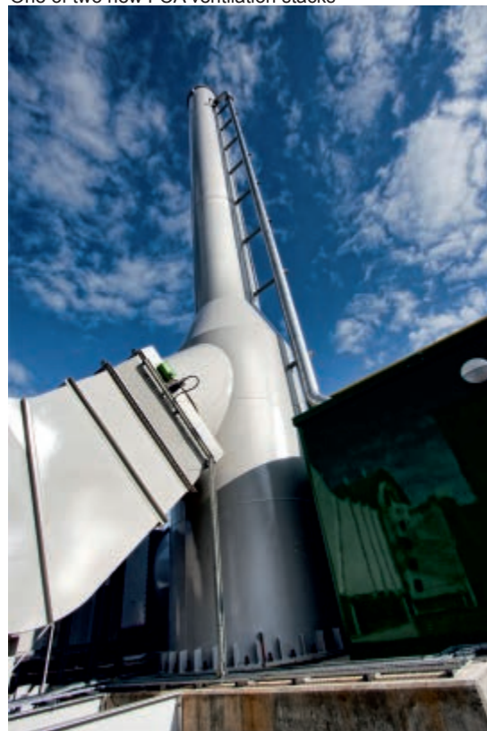
One of two new FCA ventilation stacks
