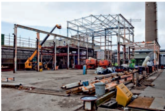
FCA building demolition in progress
