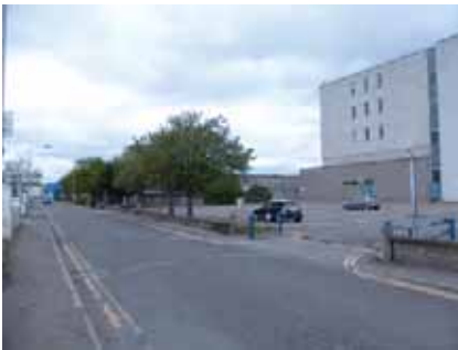
Harbour Road showing former Inverness College UHI campus.
