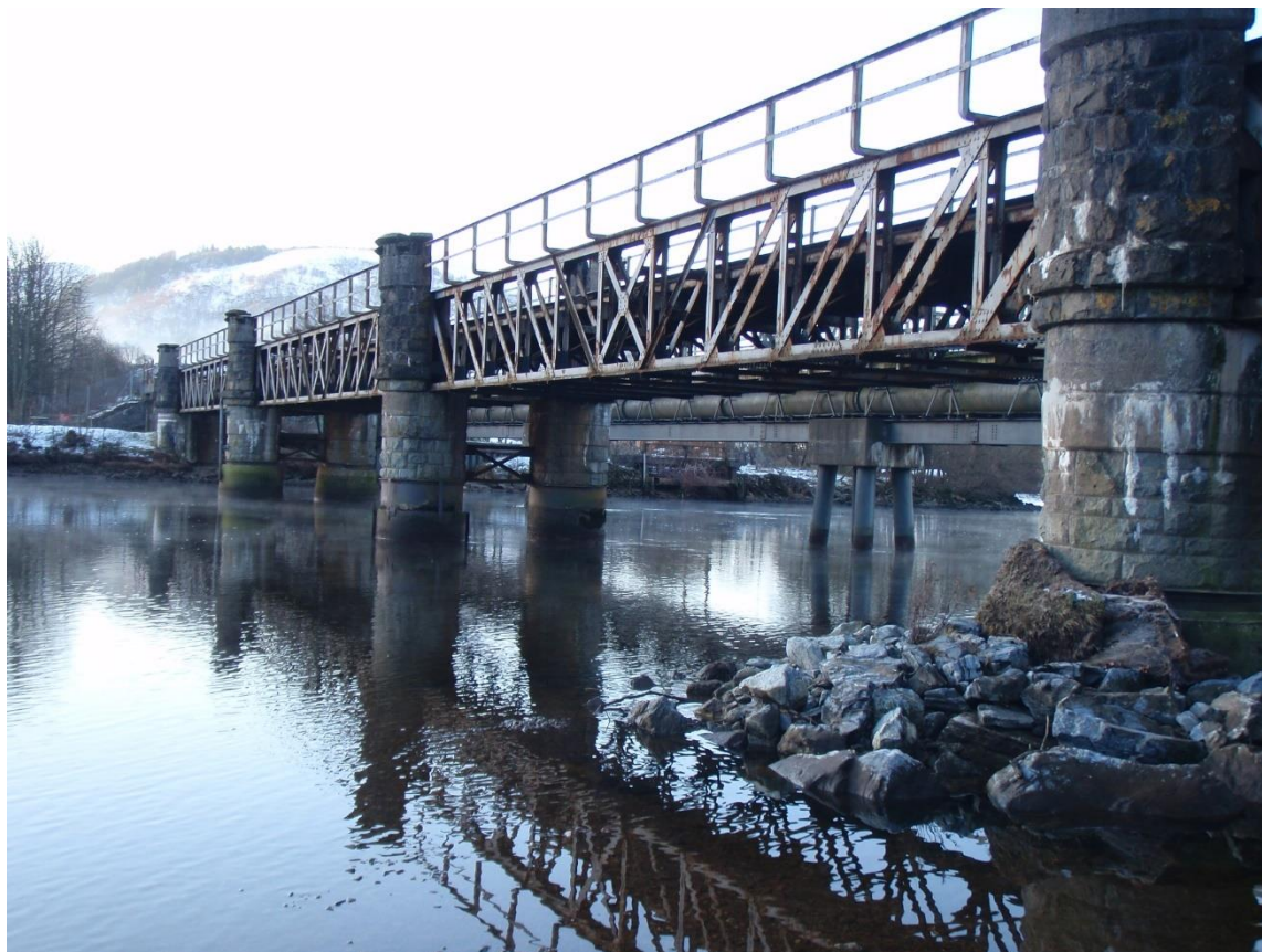
Figure 3-6: The railway and footbridge downstream (taken from right bank)
