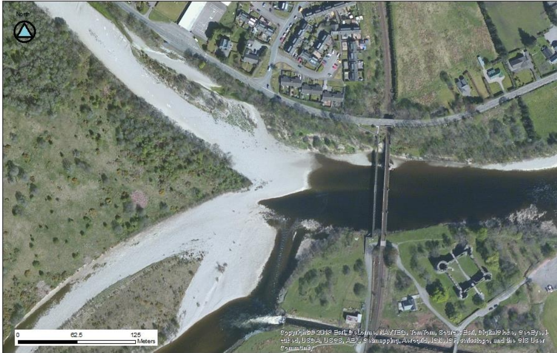
Figure 2-2: Aerial view of channel split downstream of foot and rail bridge
