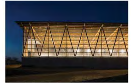
Waste facility, Lannon-Tregor, Francois Dantart
