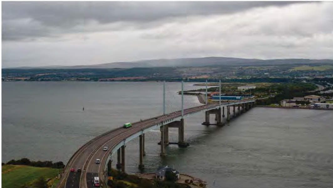
Aerial view from behind kessock bridge
