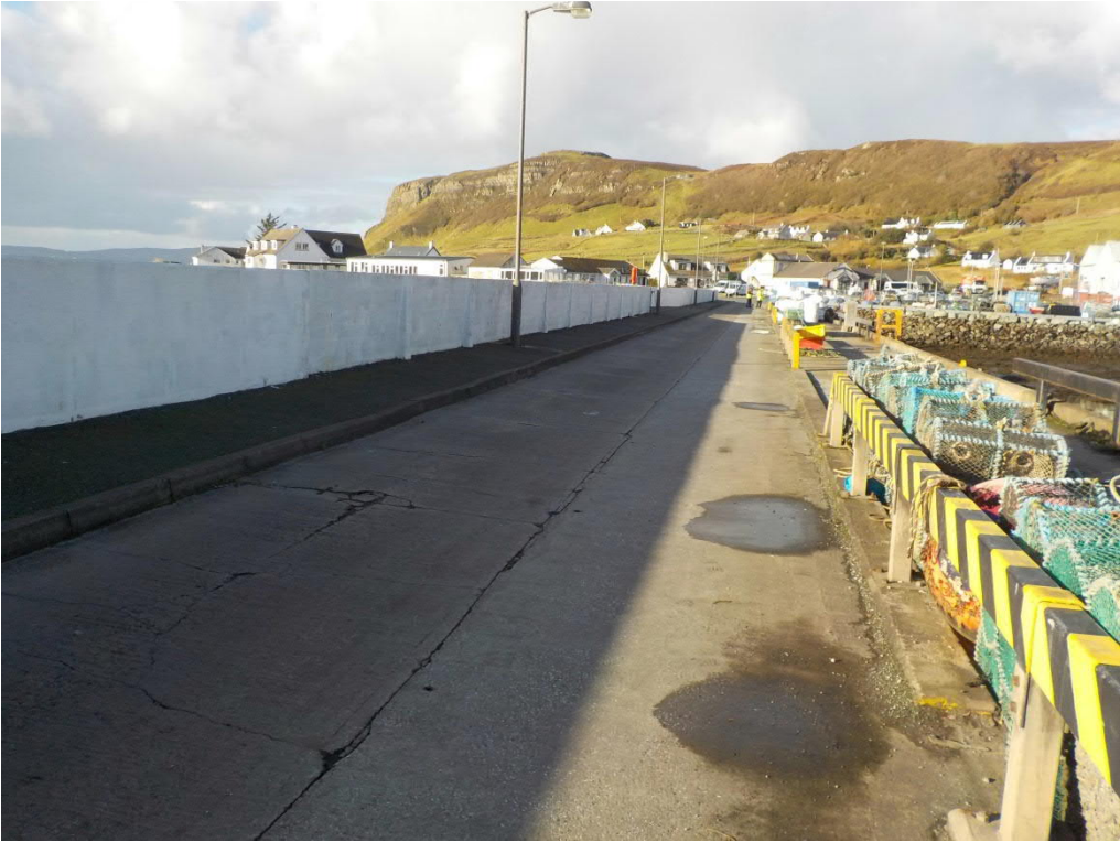
Approachway Structure Looking Back to the Marshalling Area
