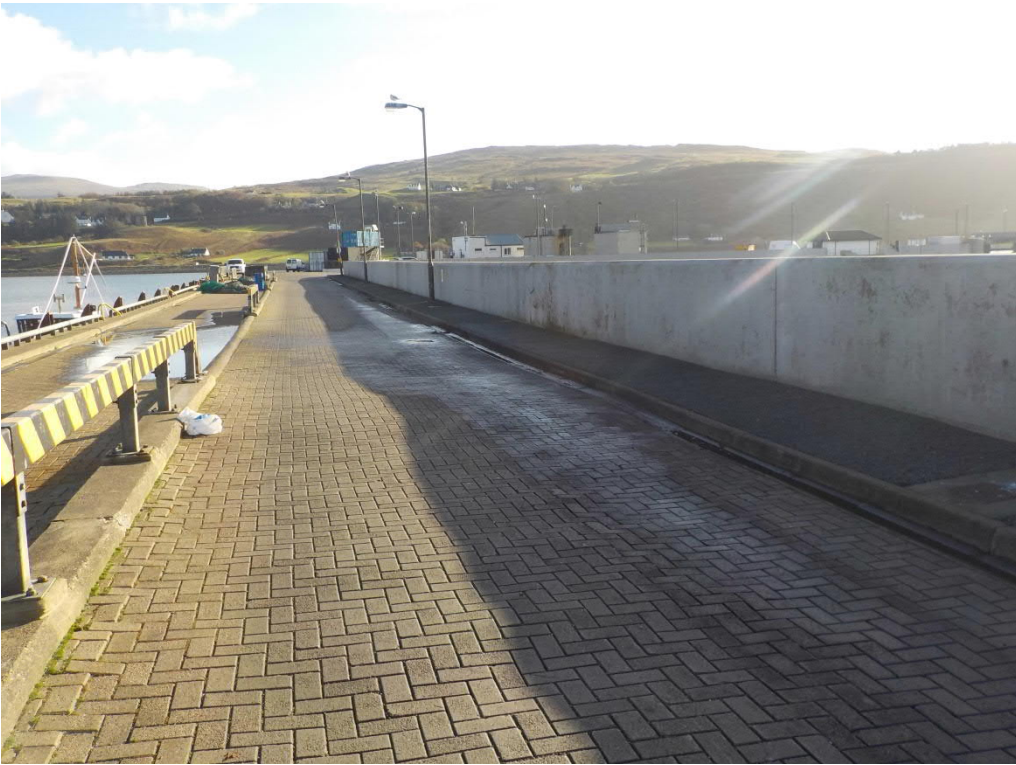
Approachway Structure Looking Towards Linkspan and Berthing Structure
