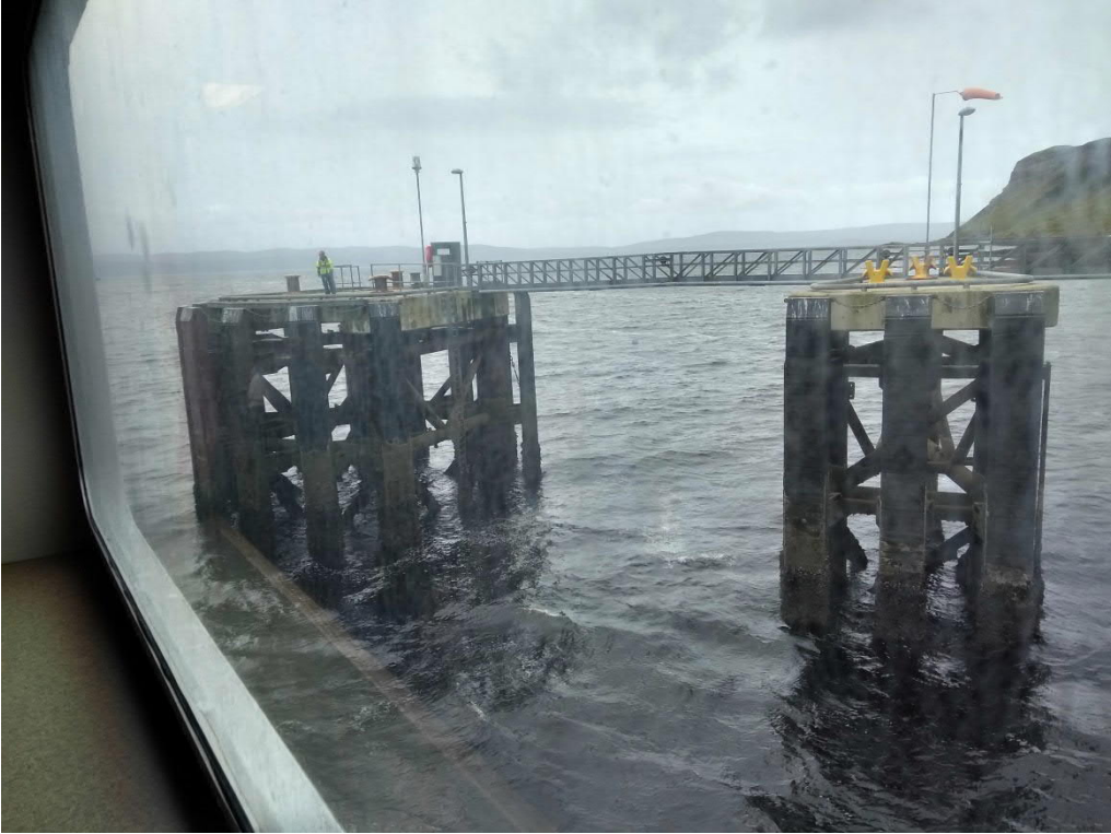
Inner and Outer Berthing Dolphins
