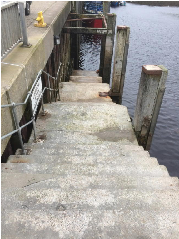
Boatsteps at Approachway
