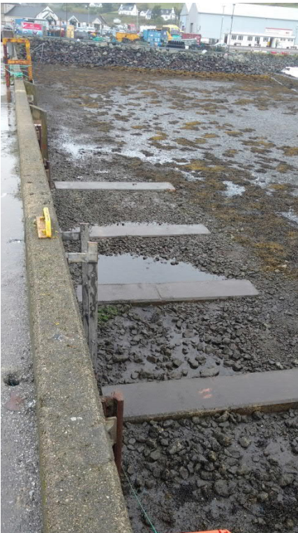
Looking From Approachway towards Fisherman's Compound and Marshalling Area
