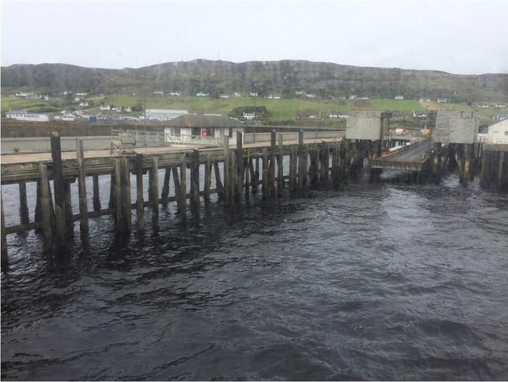
Ferry Berthing Structure and Linkspan
