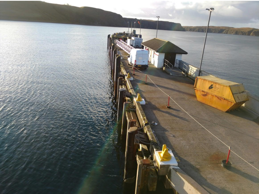
Ferry Berthing Structure
