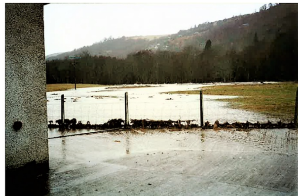
Upstream of A82 Bridge showing flooding pattern in field.
