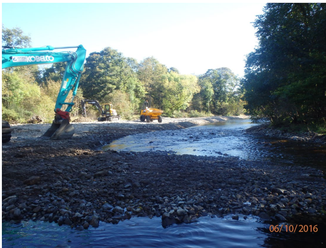
Figure 2-3 - Dredging Works to River Enrick, 2016
