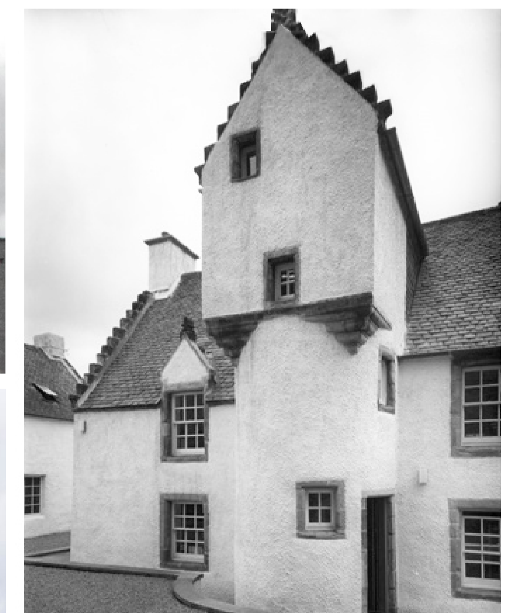
Inverness' oldest building, Abertarf House remains today, with heavy masonry walls and signature stepped gable ends.
