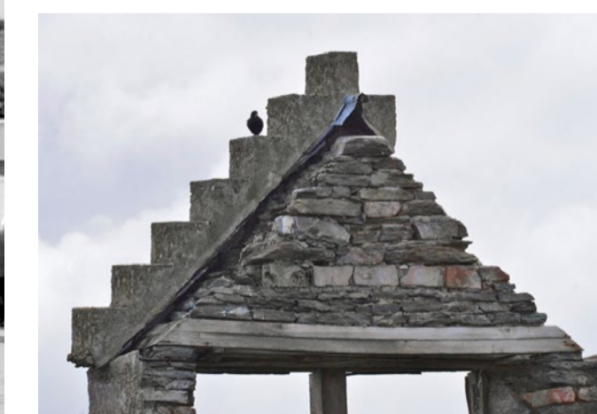
The crow-stepped gable has become synonymous with a Scottish medieval style of architecture
