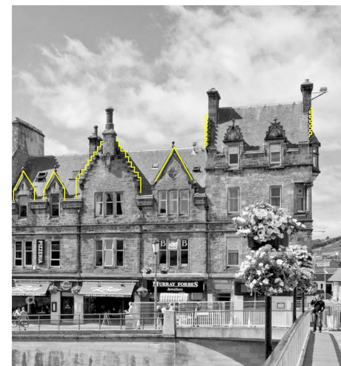
The waterfront in Inverness city centre, shows the Danish architectural influences with the stepped gables and figurative facade features.
