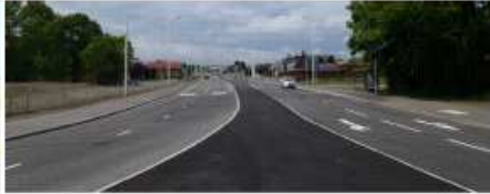
Chapel Level dual carriageway construction
