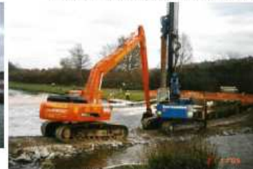
Caledonian Canal cut off using bund and sheet pile wall for dewatering
