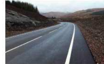
A82 Crafnalrich bypass road construction
