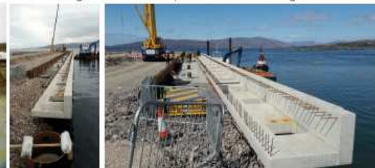
KyleakIn pier concrete edge beam construction
