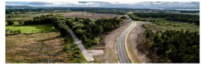
Clephanton Bends Road Construction
