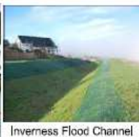
Inverness Flood Channel geotextiles and seeding
