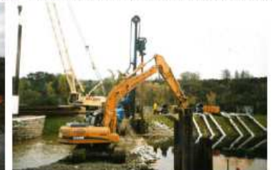
Caledonian Canal cut off using bund and sheet pile wall for dewatering
