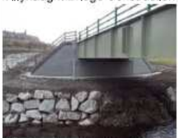
Tillynaught Bridge Construction
