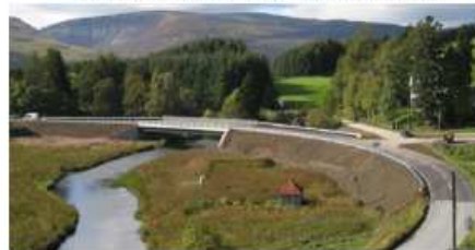
Amurlee Bridge Replacement
