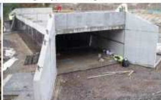
Inverness Flood Channel box culvert construction including management of services
