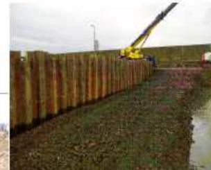
Macduff harbour bund & piling cut off wall
