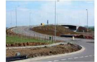
A77 Symington Road and bridge construction
