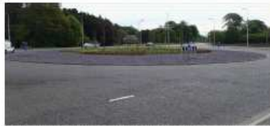
Chapel Level road & roundabout construction
