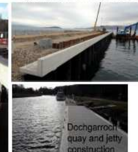
KyleakIn pier concrete edge beam construction
