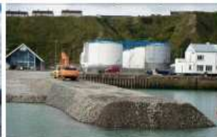
Scrabster Harbour bund construction
