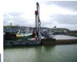
Bund and cut off piling In operational Macduff harbour
