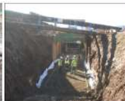
Inverness Flood Channel box culvert construction including management of services
