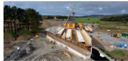
A75 Dunragit Bypass Bridge construction
