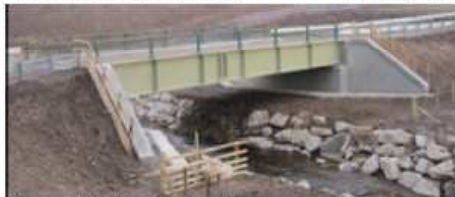
Tillynaught Bridge Construction
