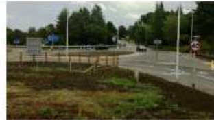
M876 Glenbervle Slip Roads and roundabout construction
