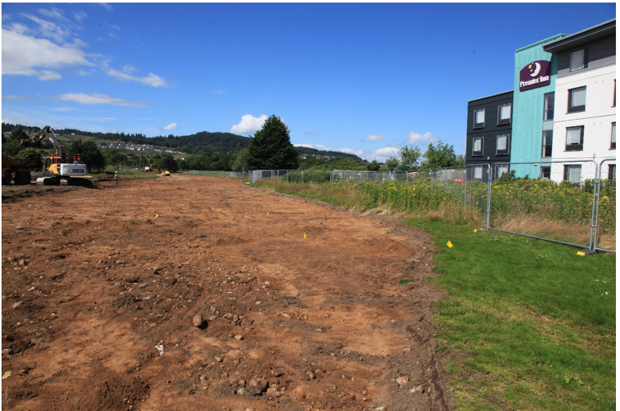
Topsoil Strip on the New General Booth Rd
