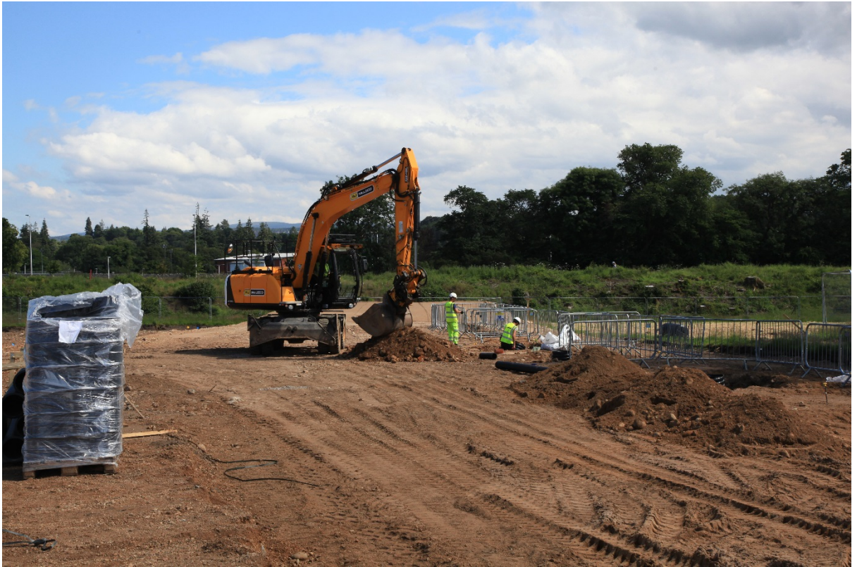
Drainage installation on the new canal access
