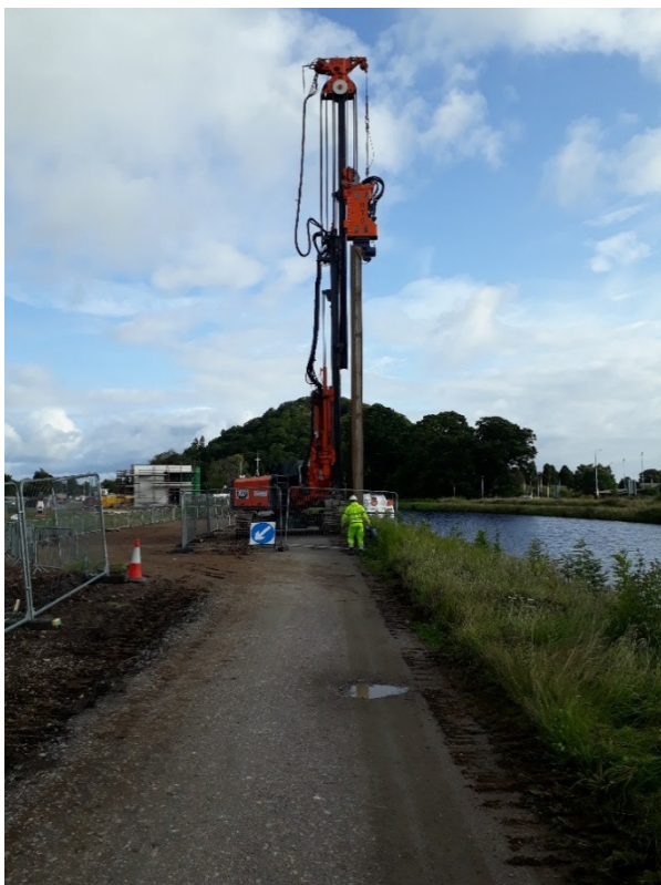
Piling Rig installing piles on towpath
