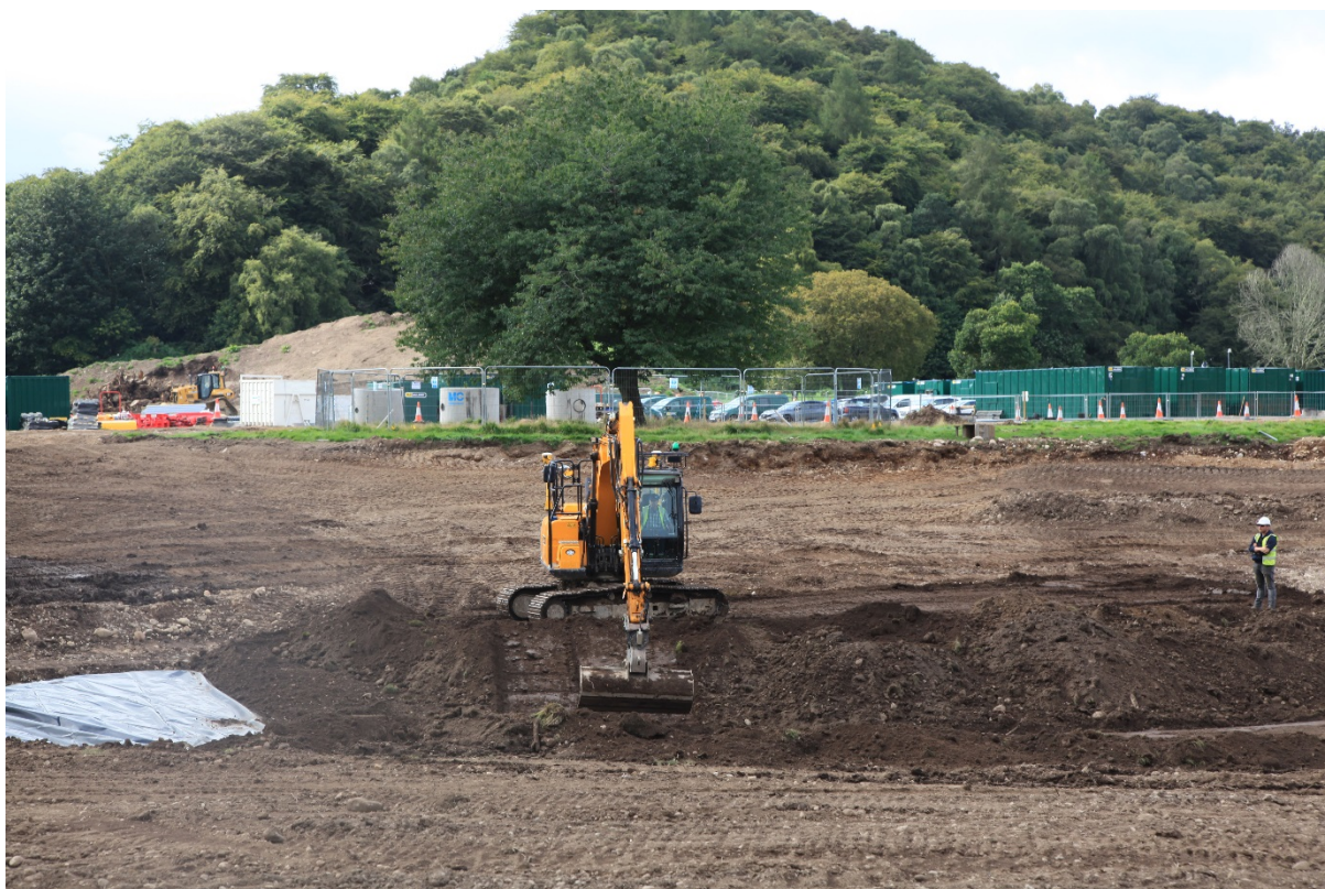
Placing liner and shaping the SUDS pond using GPS Machine Control
