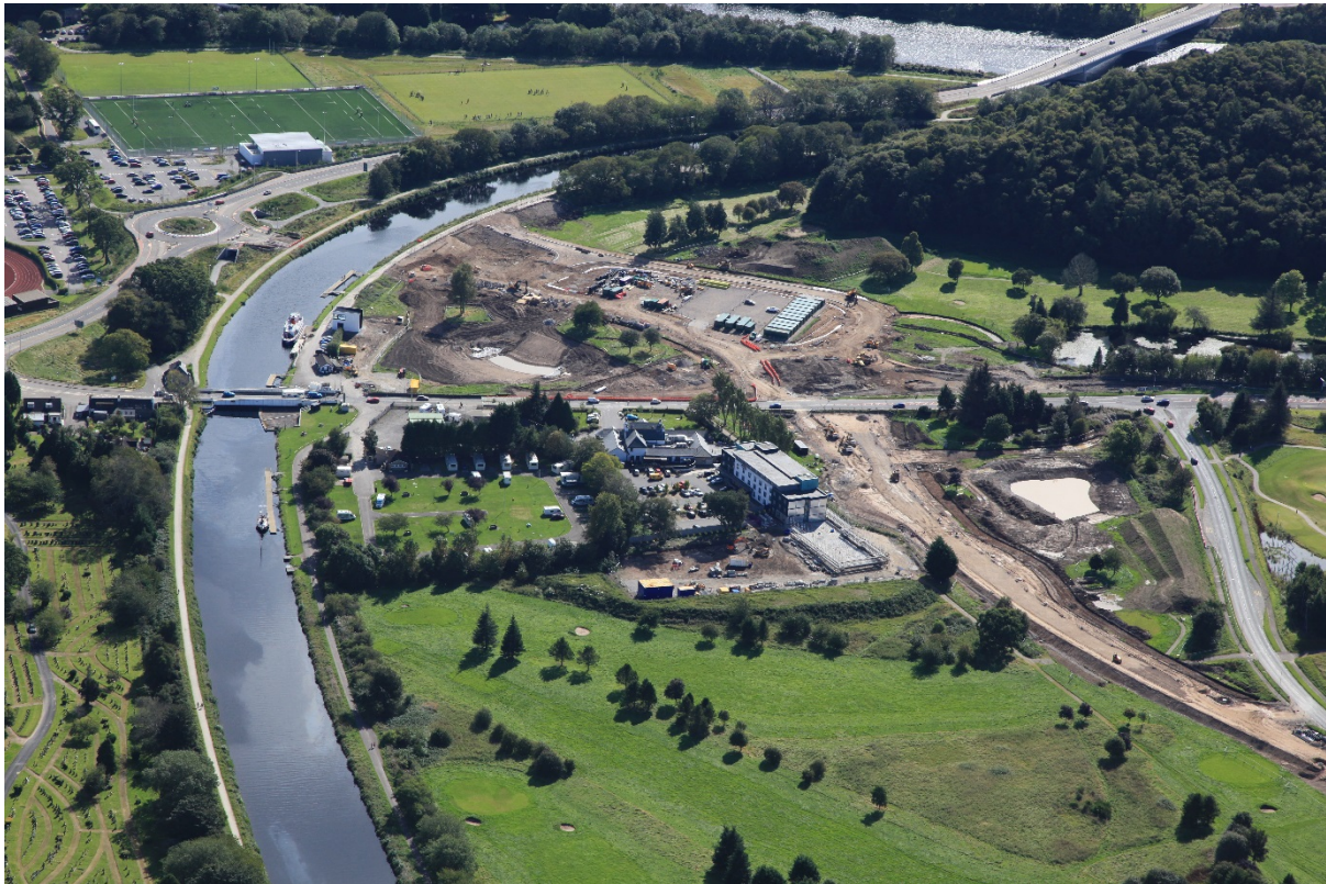
Aerial view of the site
