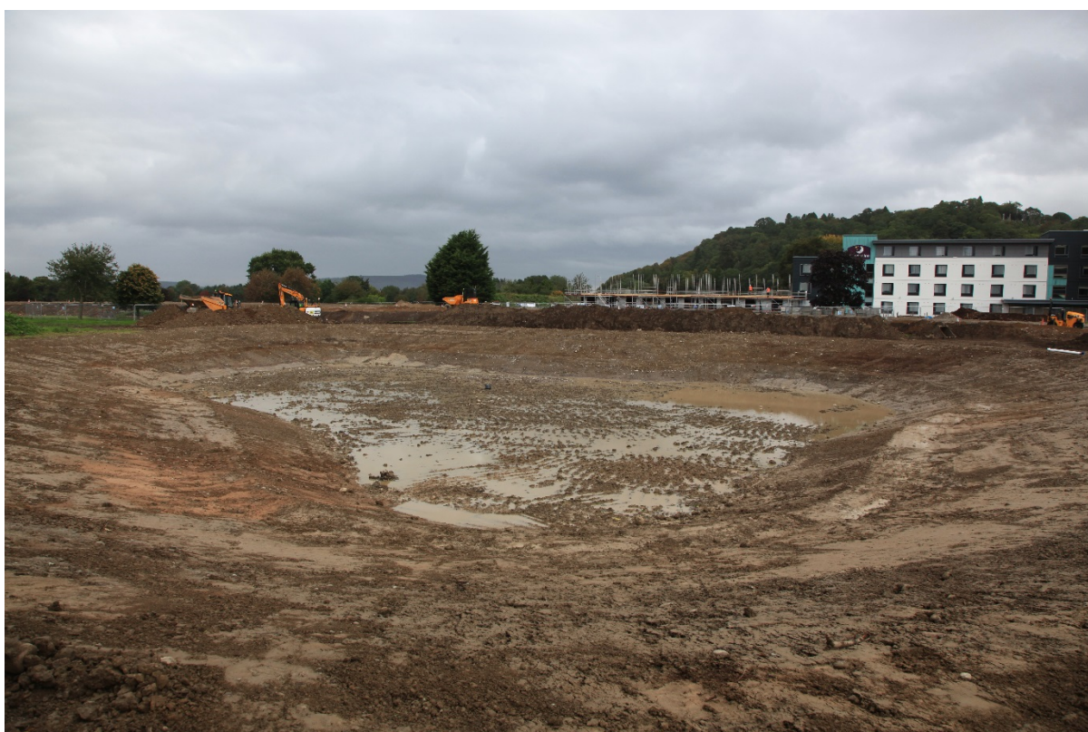
Formation of new SUDS pond to North of A82 – awaiting liner
