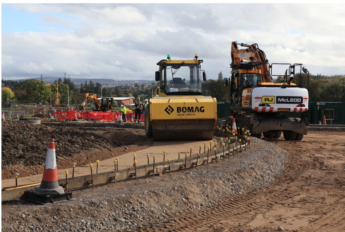
Installing kerb logs on the new roundabout
