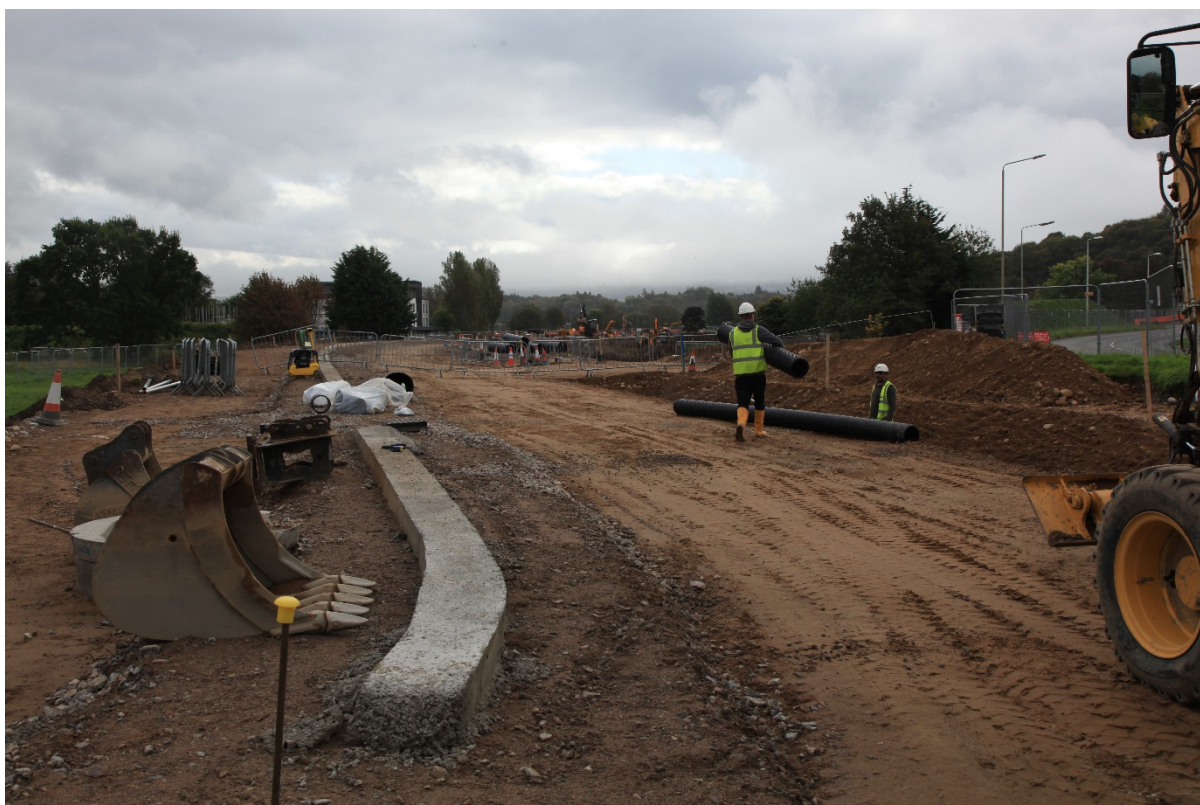
Installing drainage and kerb logs on the new General Booth Road
