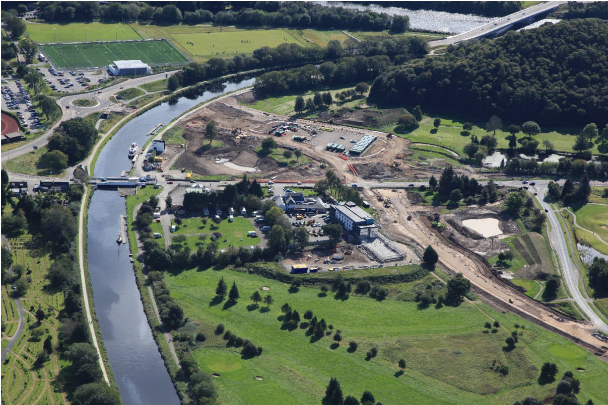
Aerial photo of the site from the North
