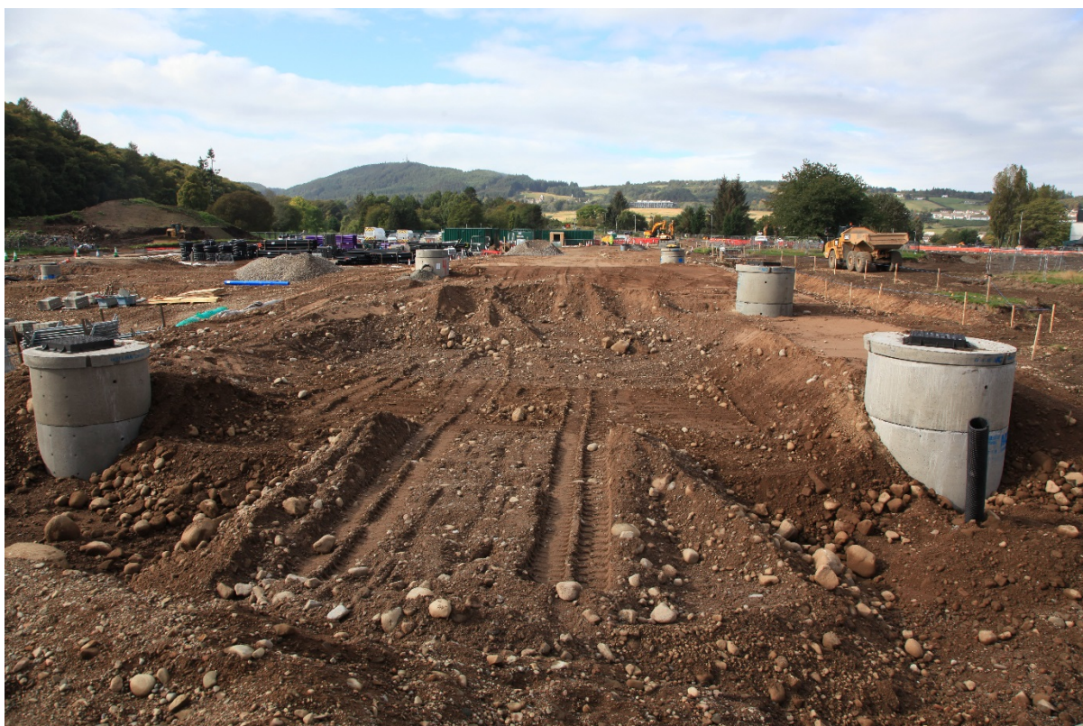
Installation of catchpits on new bridge access
