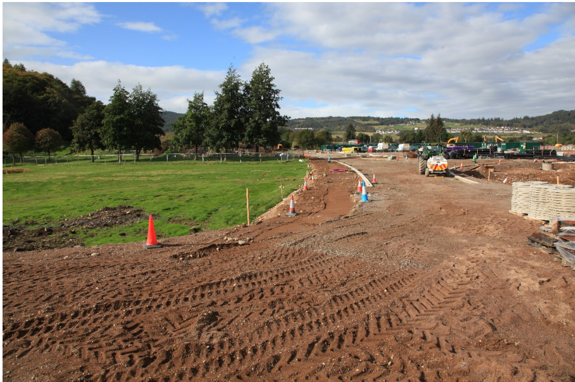
Kerb installation on the new canal access
