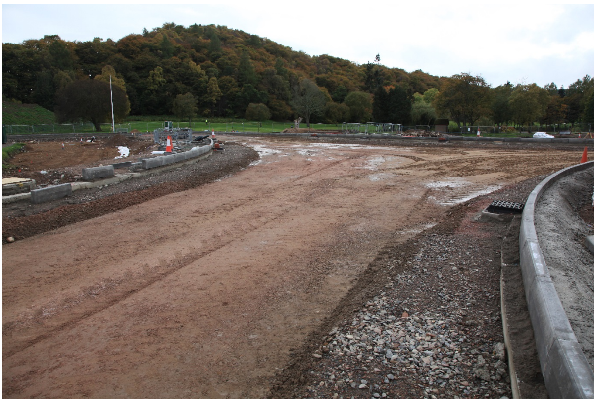
Kerbs on the new roundabout
