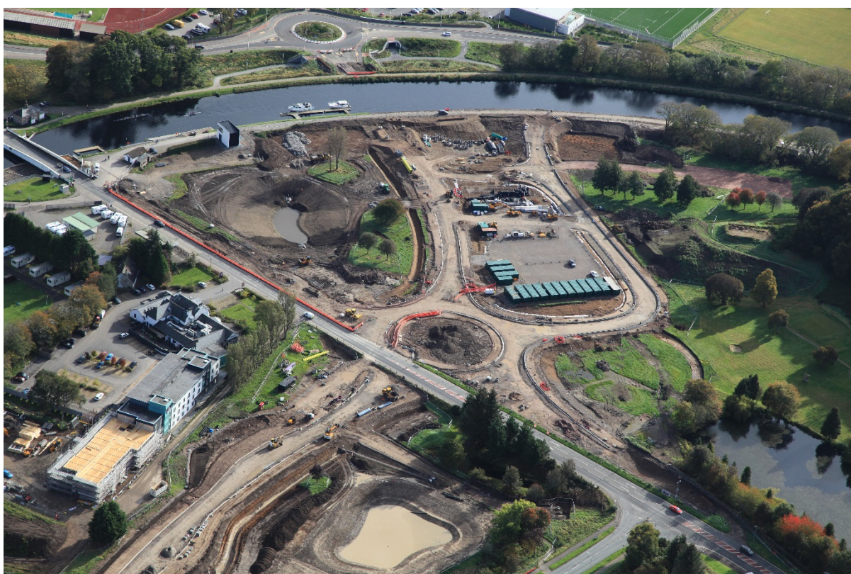
Aerial photo of the site from the North East
