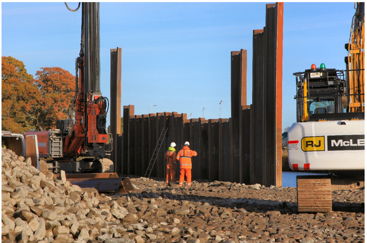
Driving sheet piles on wharf
