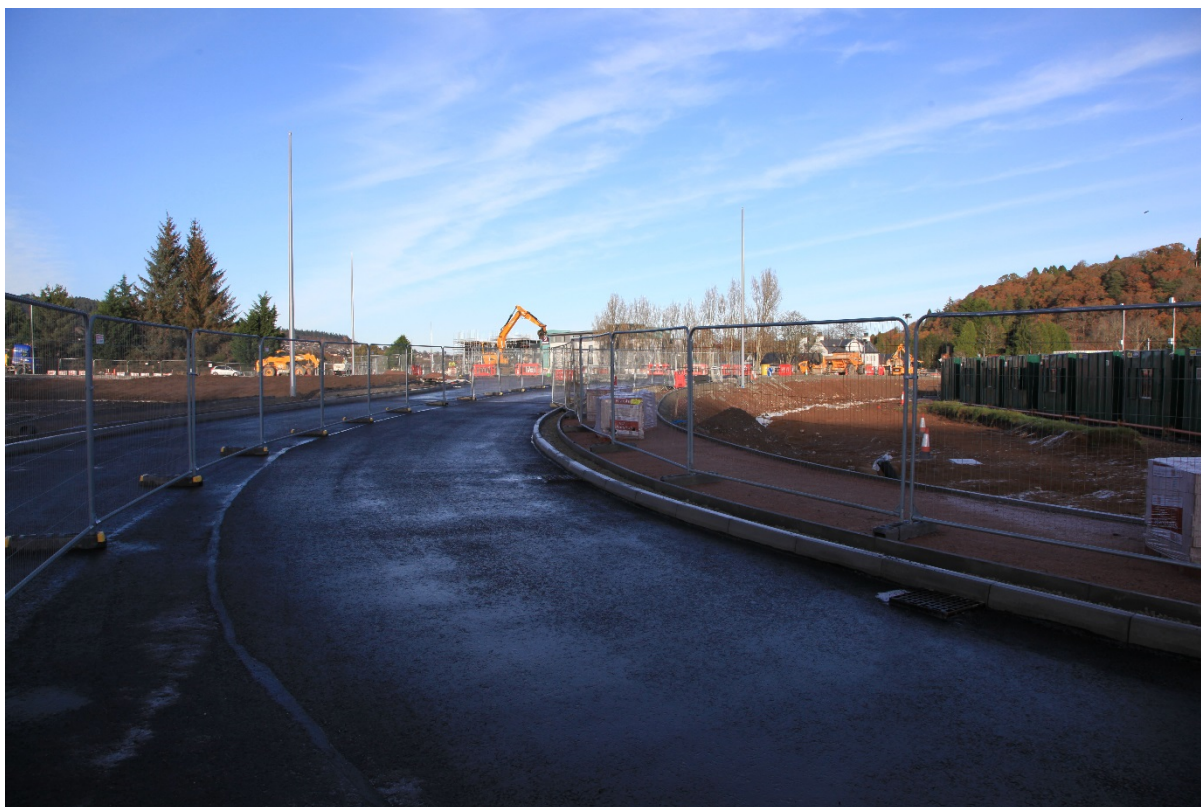
Kerbs & Surfacing on the canal access
