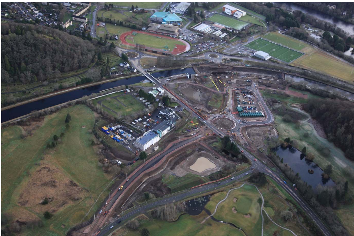
General Booth Road and the new roundabout on the A82
