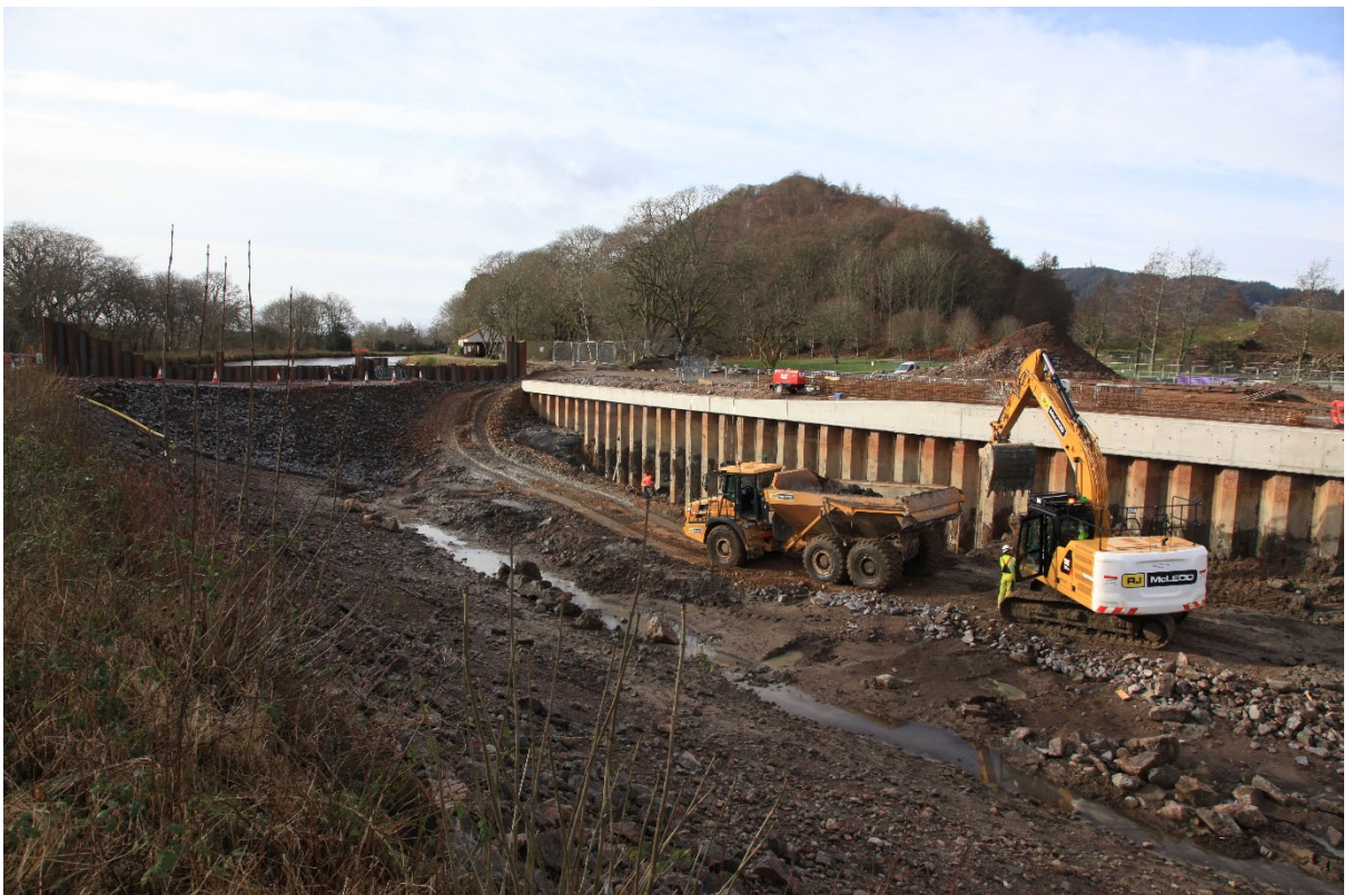
Excavation of canal invert along the front of the new wharf
