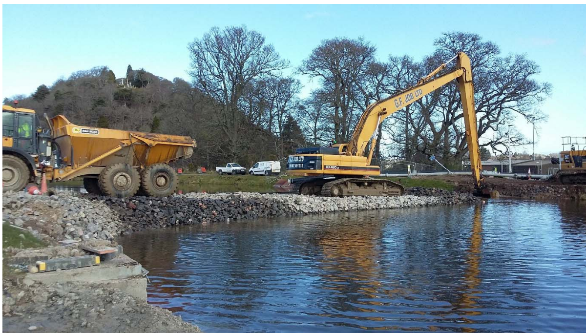
Removal of the North Stone Dam with Long Reach Excavator
