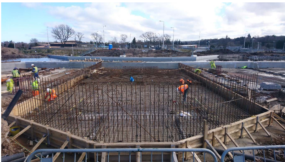
Swing Bridge apron reinforcing.
