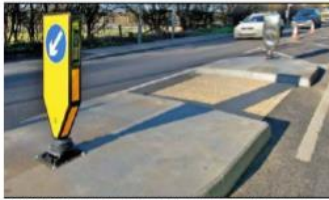
Ref 03 - BUCK ROAD (small built in bollard and line to form cycle lane and pedestrian crossing point leading to concrete footway)
