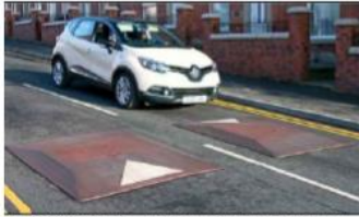
Ref 03 - (S)D EVANTON ROAD (small speed hump in proximity of wall and pedestrian crossing point)
