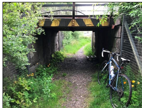
Figure 4-98 - Greenspace Bounded by West Highland Railway Line, Fern Court and Moor Road [2]
