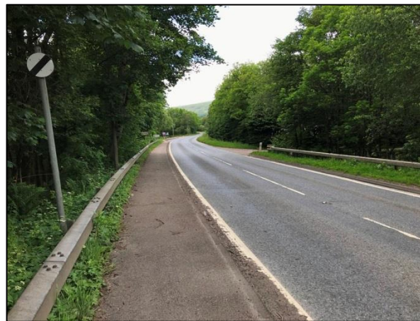
Figure 4-69 - A830 West of Banavie Rail Station [4]
