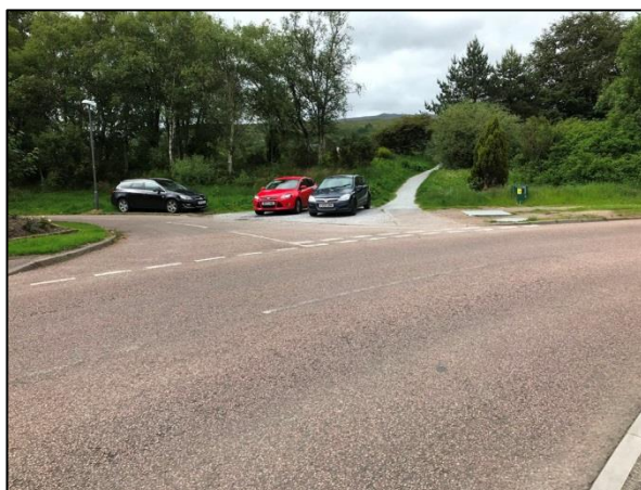
Figure 4-91 - B8006 Kilmallie Road [3]
