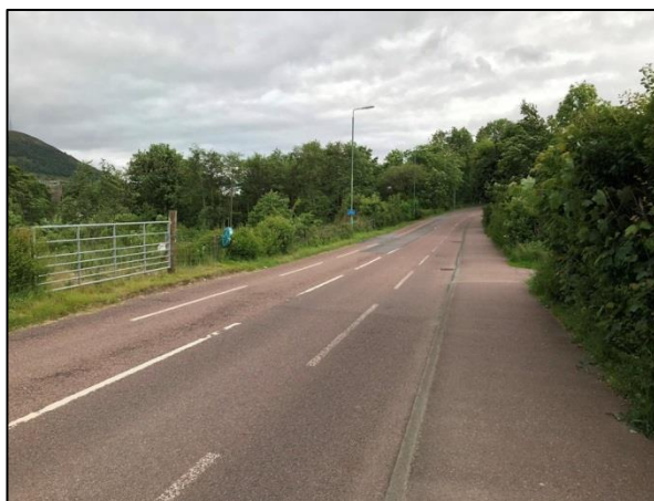
Figure 4-89 - B8006 Kilmallie Road [1]
