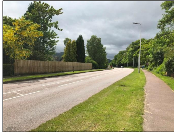
Figure 4-67 - A830 West of Banavie Rail Station [2]
