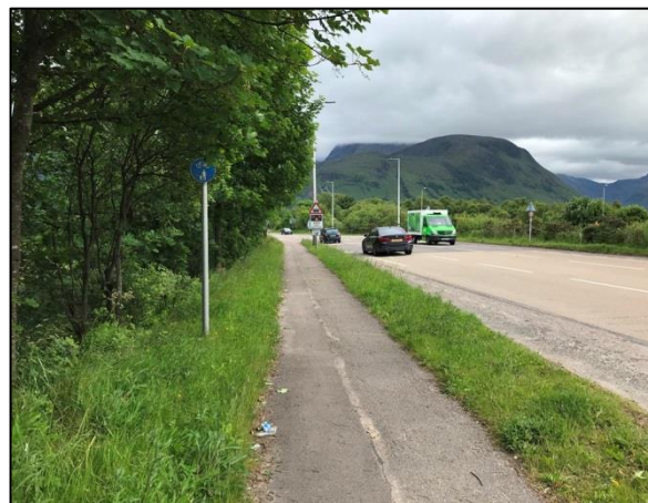
Figure 3-25 - Shared Use Footway, A830
