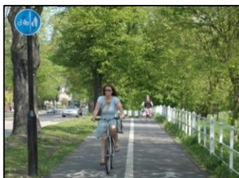
Figure 4-7 - Shared Use Footway/Cycleway with Segregation, York
