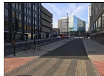
Figure 4-9 - Dual Carriageway Converted to Single Carriageway with Cycleway, Newcastle
