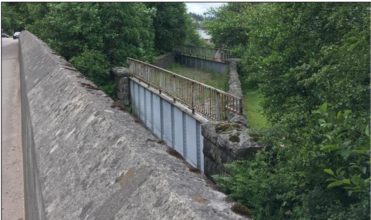
Figure 4-58 - A82 North Road from River Nevis Bridge to Fort William Retail Park [3]
