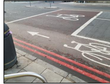
Figure 4-12 - Advanced Stop Line
