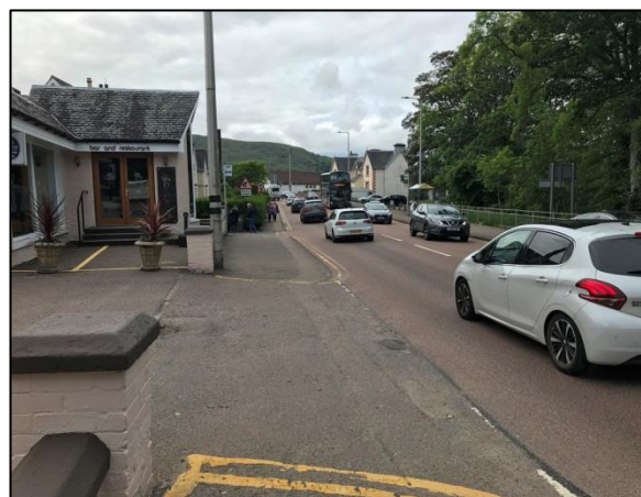
Figure 4-55 - A82 Belford Road from Old Fort / Fort William Railway Station to River Nevis Bridge [4]
