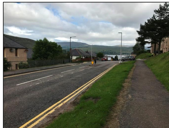
Figure 4-108 - Lundrava Road, from West End Roundabout to Lundrava Primary School [4]
