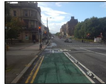
Figure 4-16 - Light Segregation
