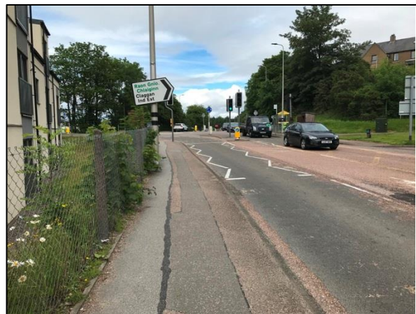
Figure 4-60 - A82 North Road from River Nevis Bridge to Fort William Retail Park [5]
