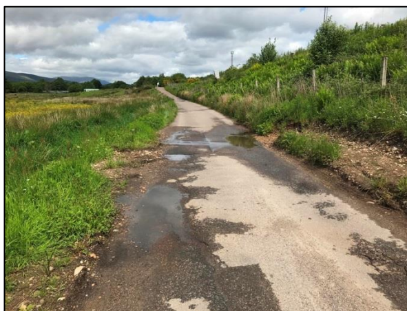
Figure 4-38 - Link from Lochiel Road to the Soldiers Bridge [1]
