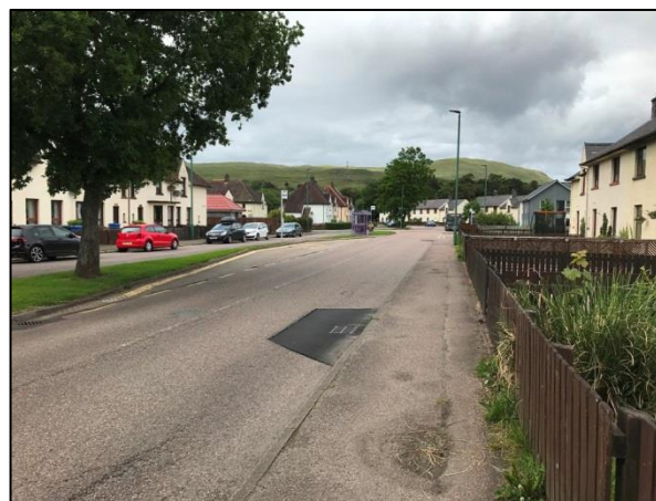
Figure 4-90 - B8006 Kilmallie Road [2]
