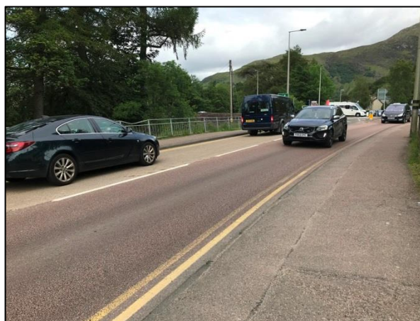
Figure 4-54 - A82 Belford Road from Old Fort / Fort William Railway Station to River Nevis Bridge [3]
