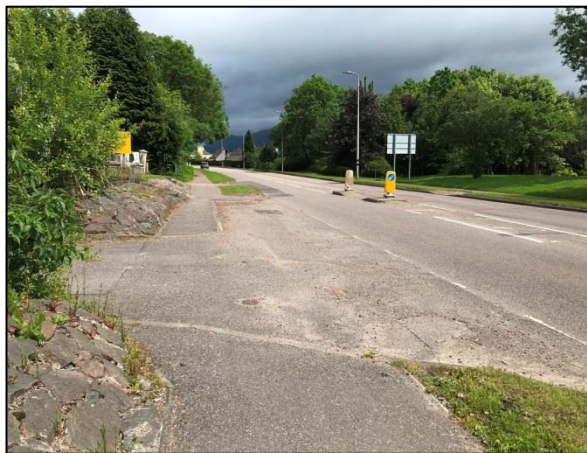
Figure 4-68 - A830 West of Banavie Rail Station [3]
