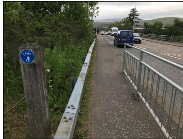
Figure 3-7 - Shared Use Footway, A830
