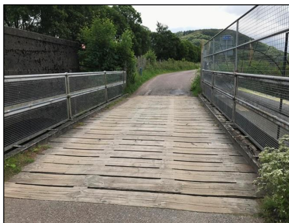
Figure 4-39 - Link from Lochiel Road to the Soldiers Bridge [2]
