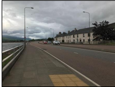
Figure 3-13 - A82, north of West End Roundabout [1]
