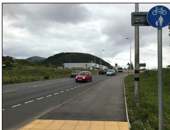
Figure 4-61 - A82 From Fort William Retail Park to Lochybridge [1]
