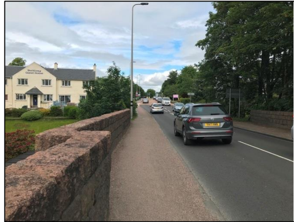
Figure 4-57 - A82 North Road from River Nevis Bridge to Fort William Retail Park [2]
