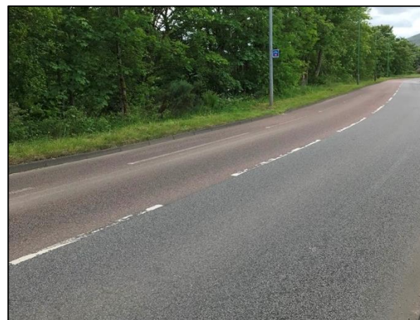
Figure 3-9 - Advisory Cycle Lanes (Kilmallie Road, at Mossfield Drive, looking south-west)
