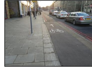
Figure 4-13 - Integration between Cycleway and Carriageway
