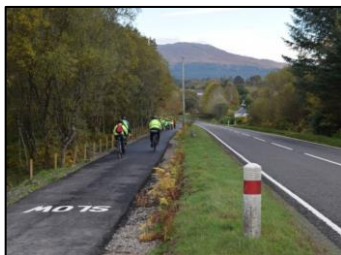
Figure 4-4 - Shared Use Footway / Cycleway, No Segregation
