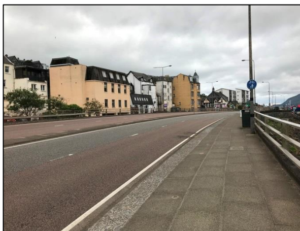
Figure 3-22 - Shared Use Footway, A82
