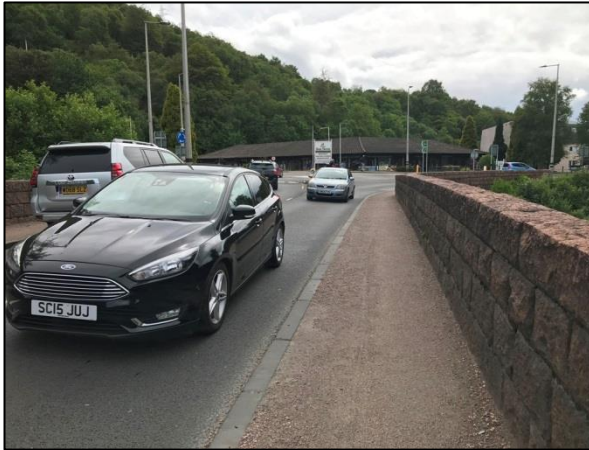
Figure 4-56 - A82 North Road from River Nevis Bridge to Fort William Retail Park [1]
