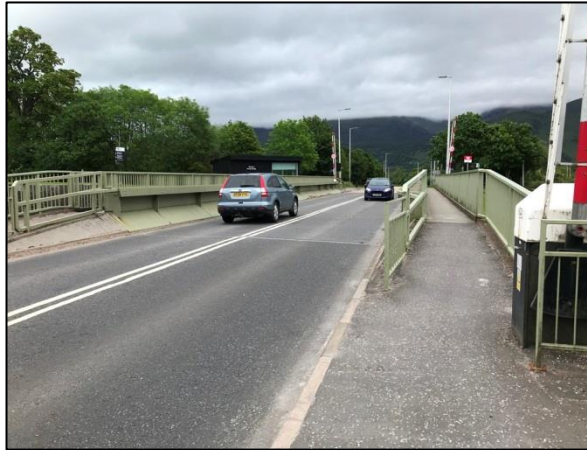
Figure 4-66 - A830 West of Banavie Rail Station [1]
