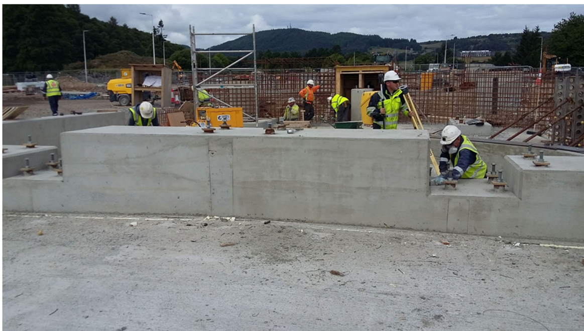
Concrete foundation for the new pivot bearing
