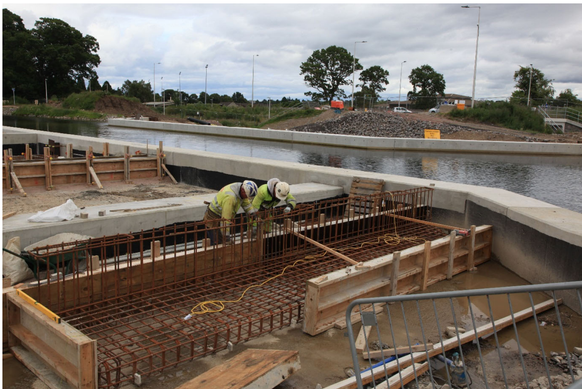
Reinforcing and shutters for retaining wall around bridge abutment
