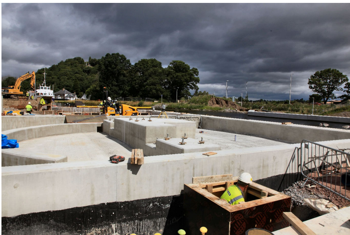
Concrete slabs and aprons for the new swing bridge
