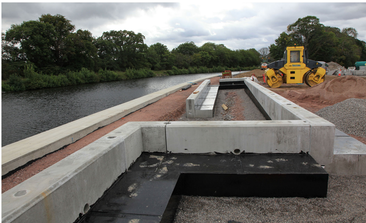
Precast retaining walls at new wharf
