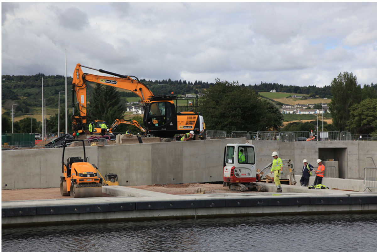
Concrete retaining walls around bridge abutment
