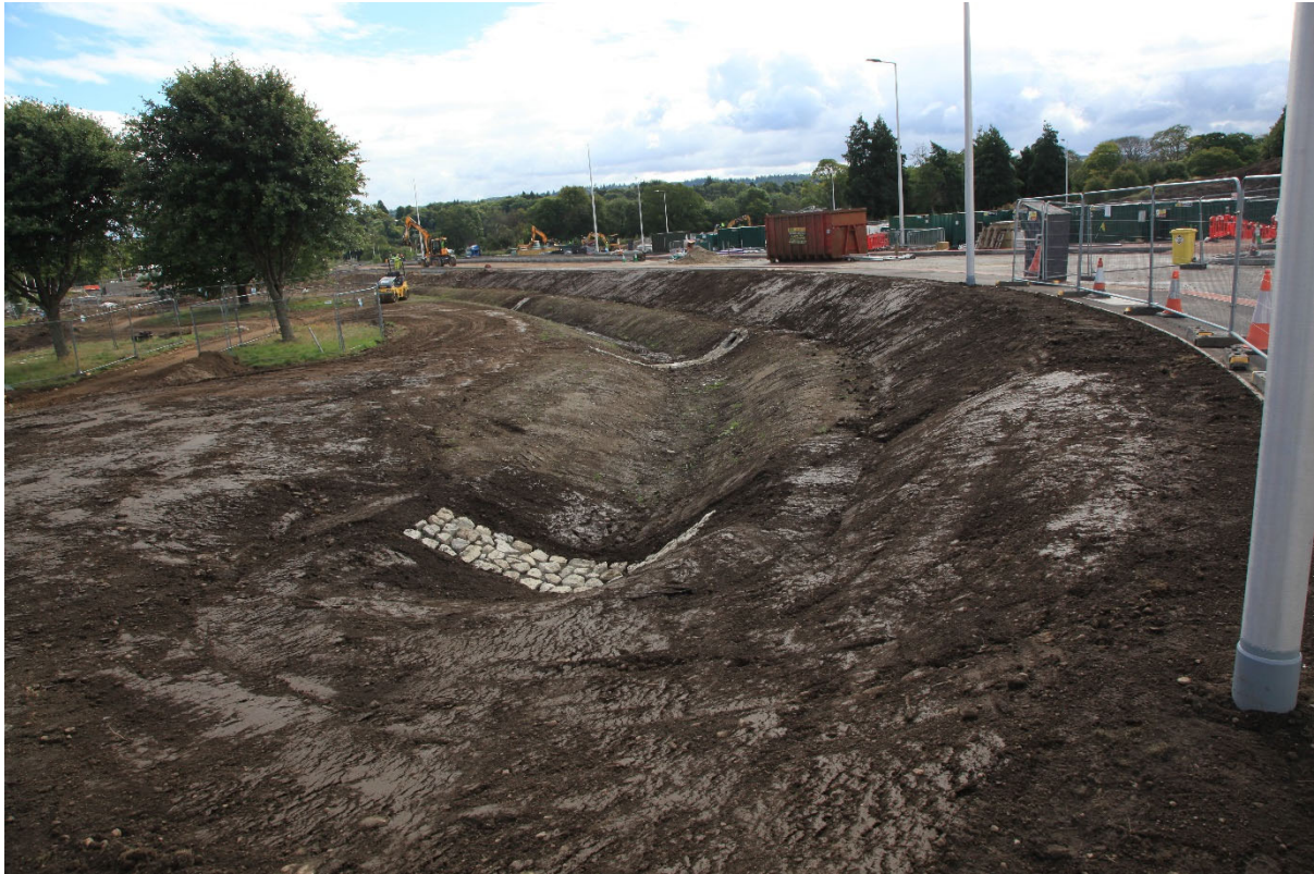
Landscaping and headwalls progressing across the site
