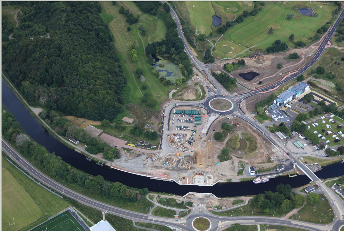
Progress Photo – Aerial Photo of the site from the east
