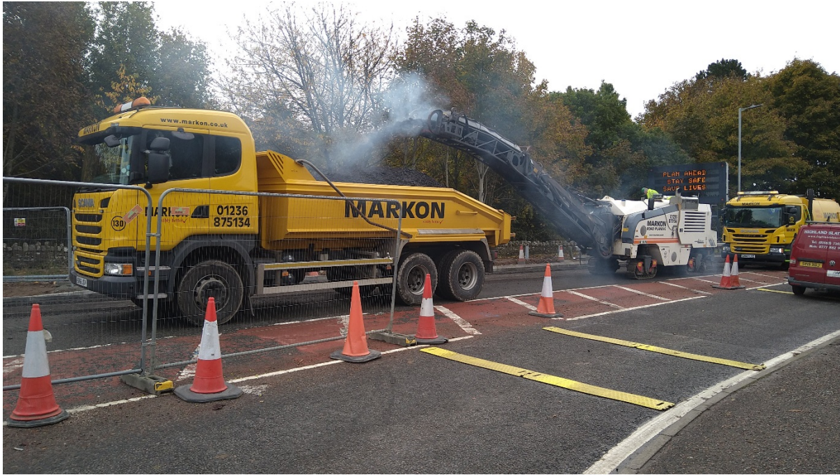
Planing out the old A82 surfacing to accommodate the new surfacing
