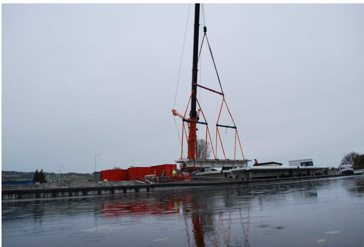
500 tonne crane lifting in the final section of the bridge
