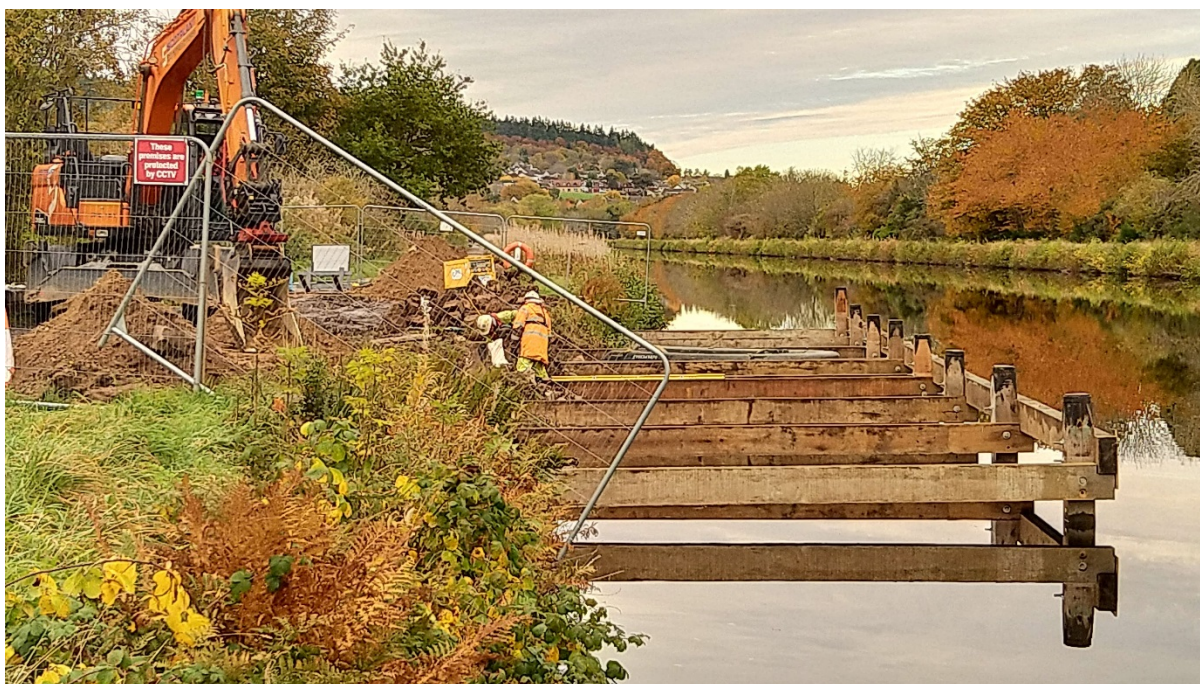
New timber jetty during construction
