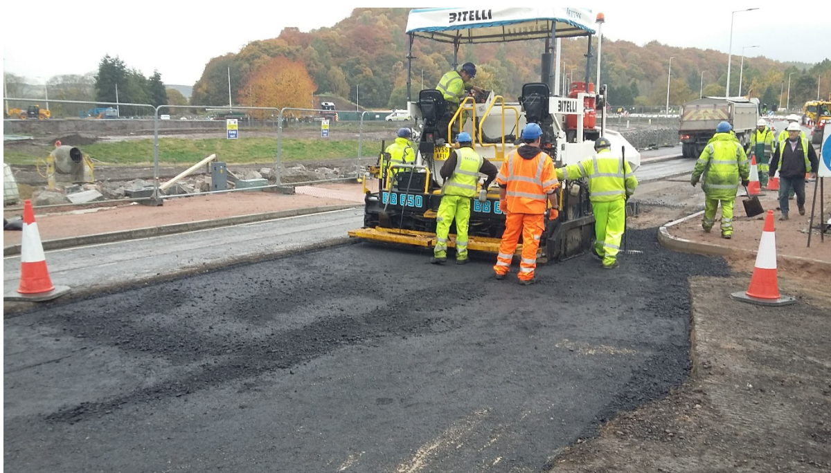
Surfacing on the A82 during one of the road closures
