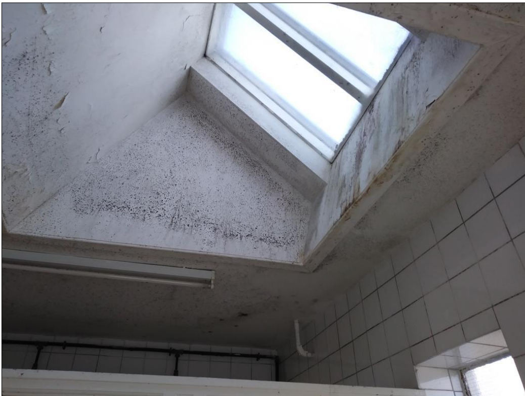
Photograph 18 – Roof Light (Female Toilet)
