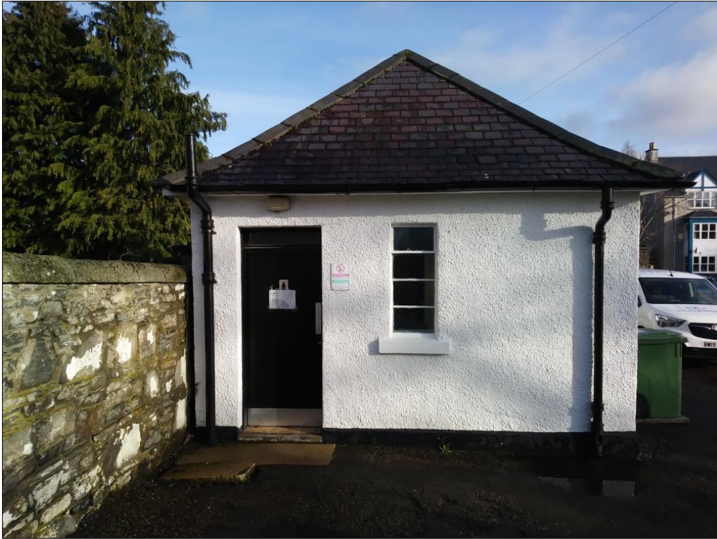
Photograph 3 – South West Elevation
