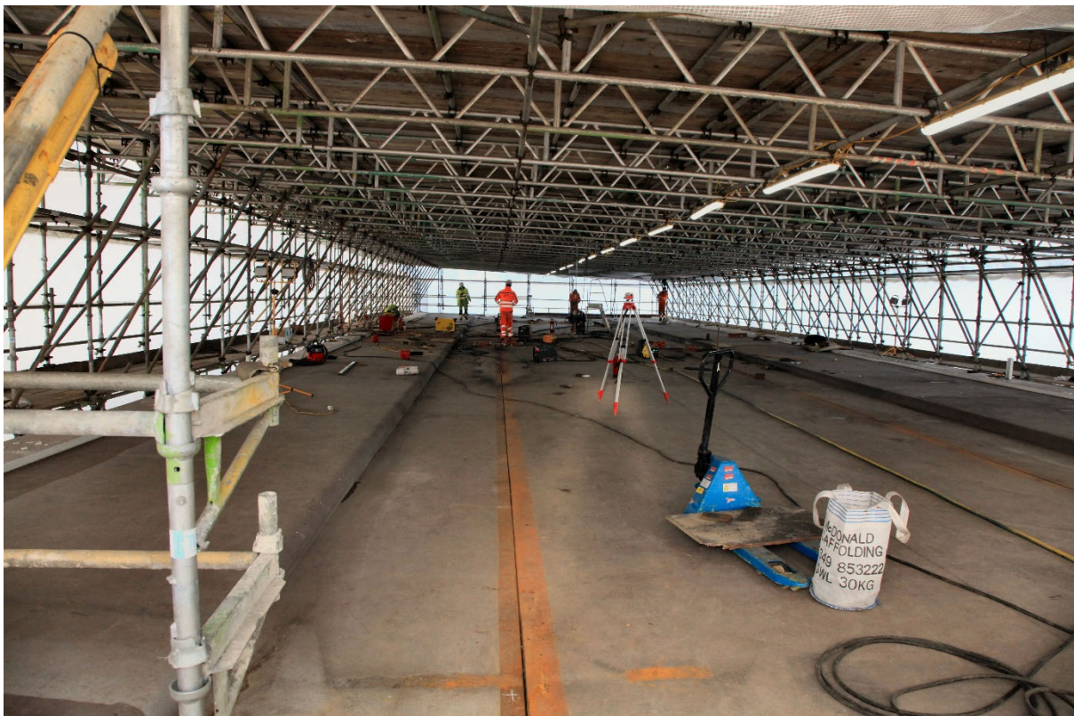
Welding of the bridge deck under cover
