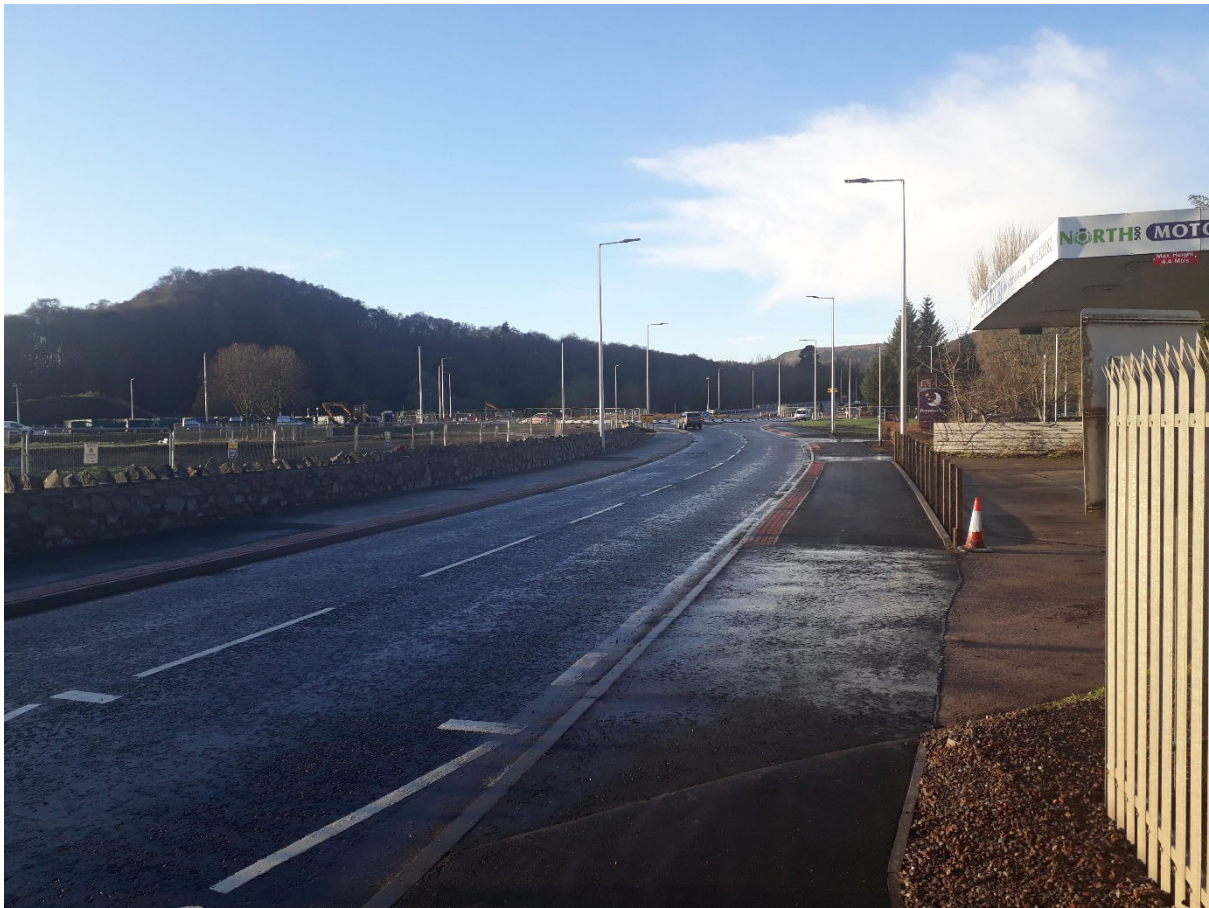
Surfacing, white lining and stone wall complete on the A82
