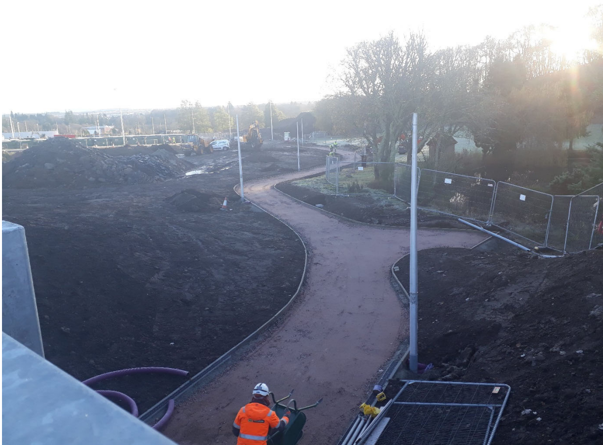
New footpath under construction into the A82 underpass
