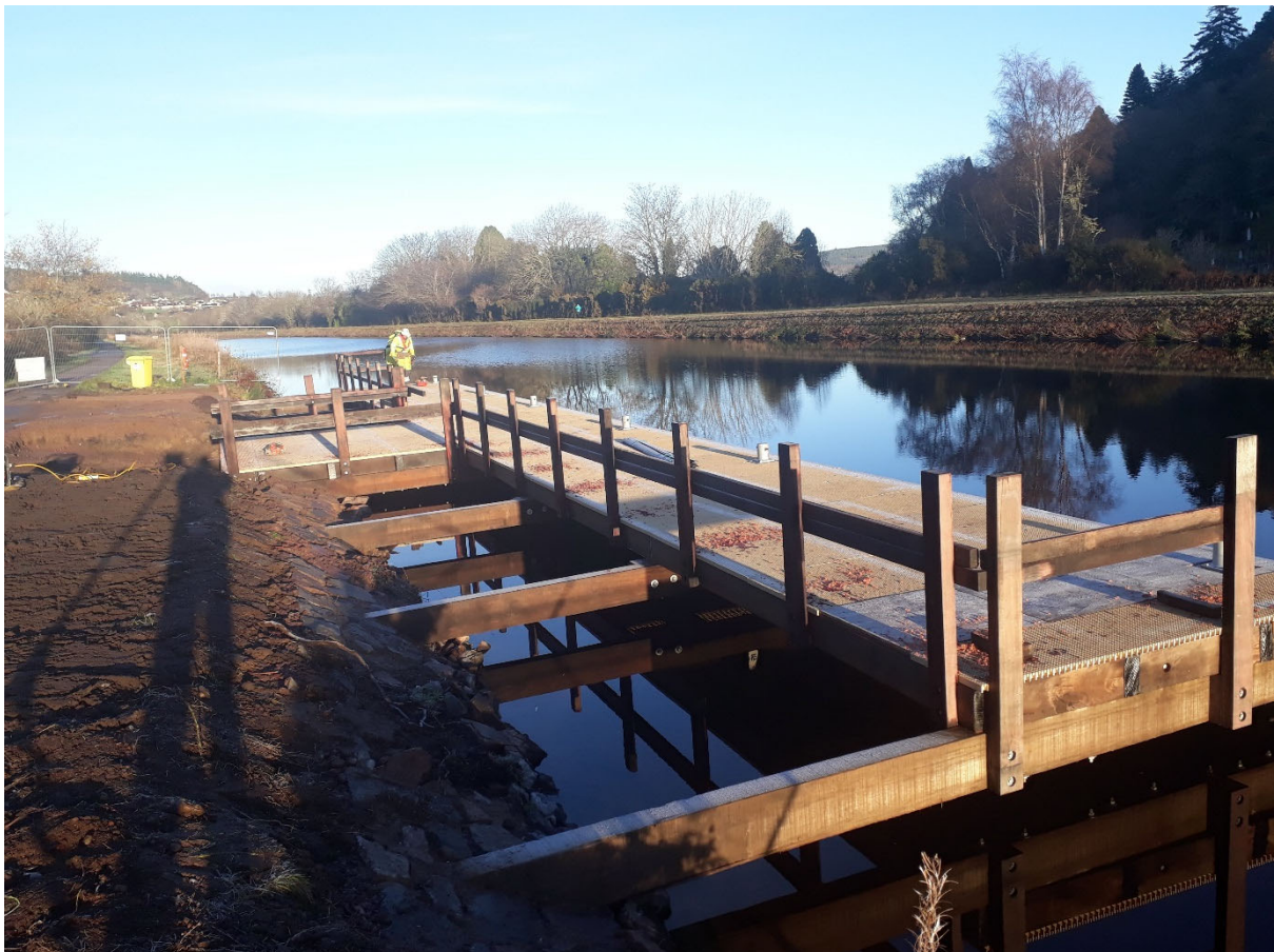
New timber jetty nearing completion
