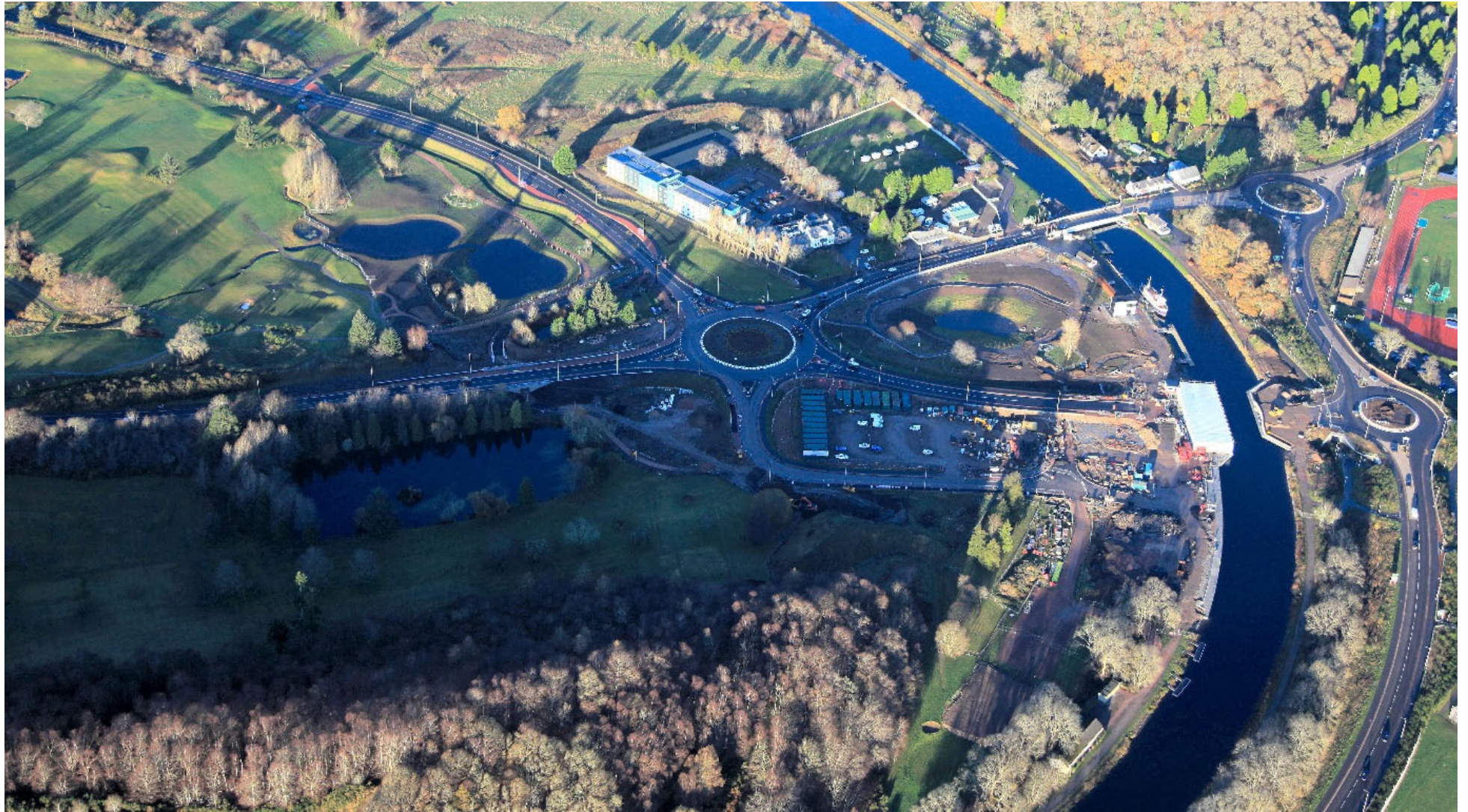
Aerial photo from the South with white bridge encapsulation and the landscaped areas beside General Booth Road
