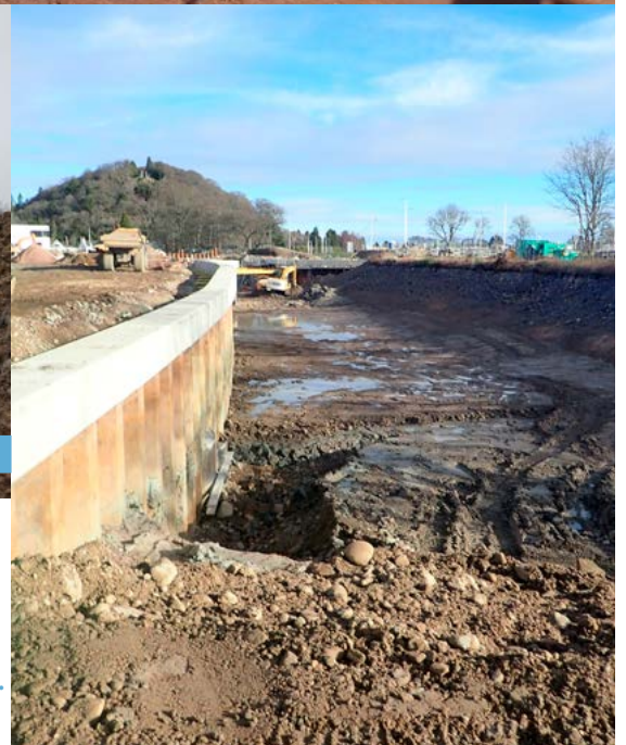
Drained section of the Canal
