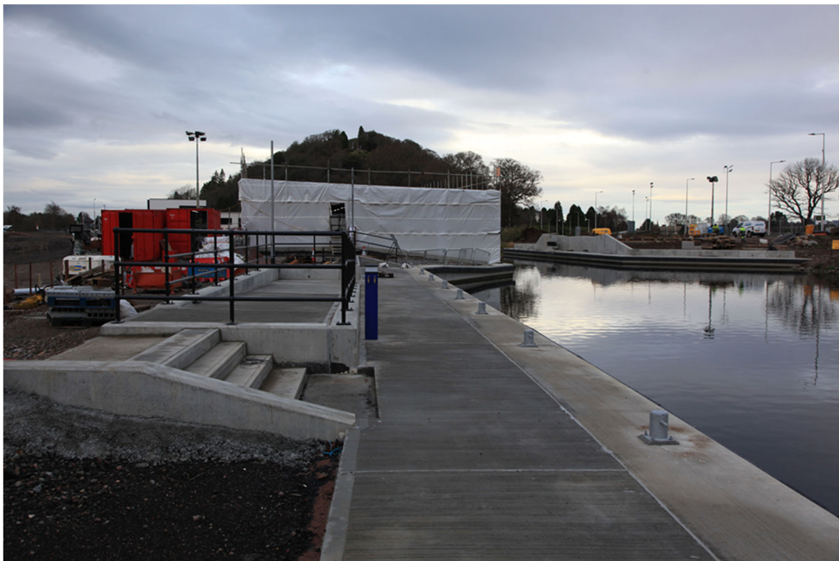
The new wharf with bollards, railings and services
