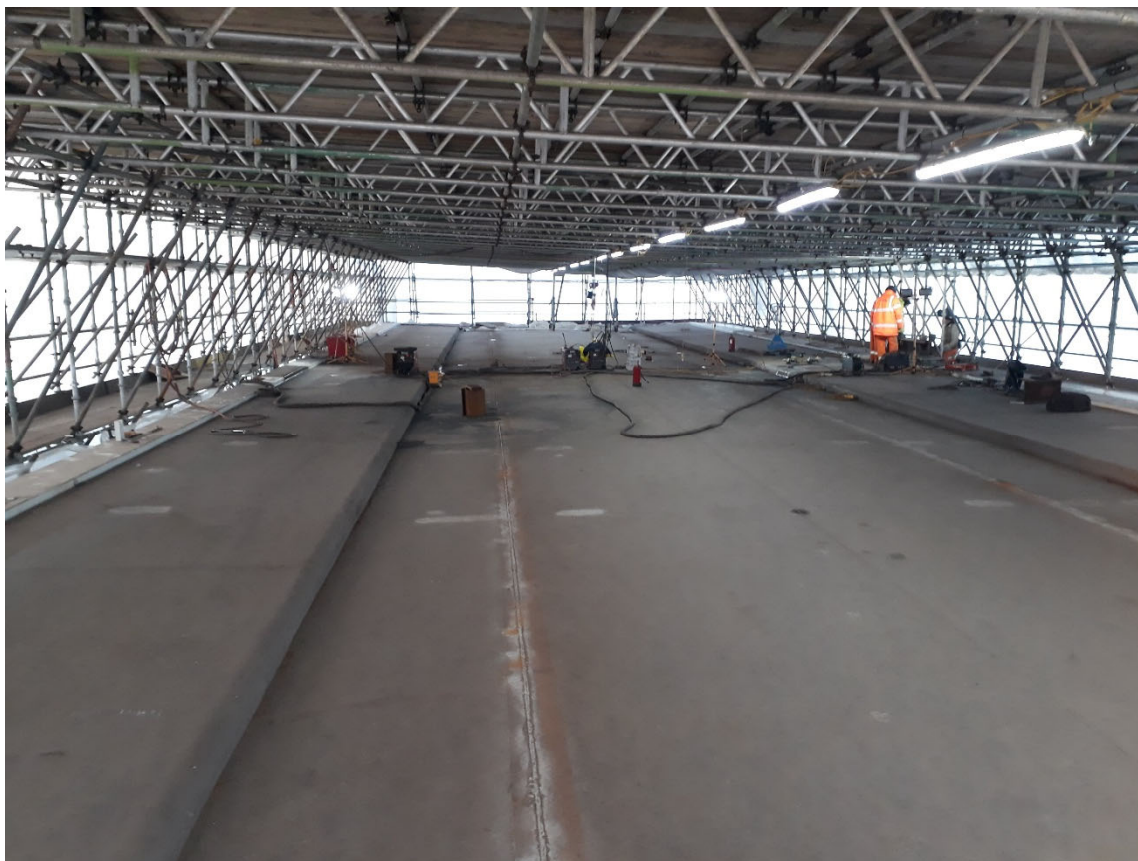
Welding the bridge sections together under the encapsulation
