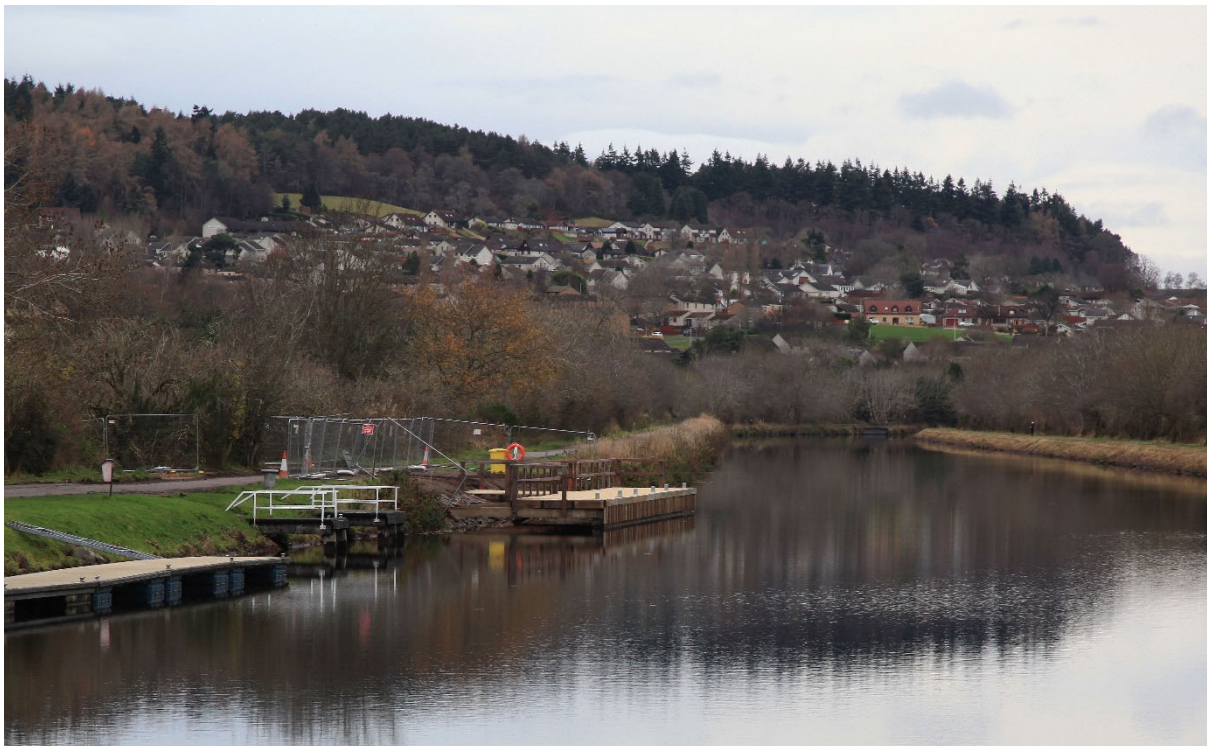
Timber jetty from Tomnahurich Bridge looking North
