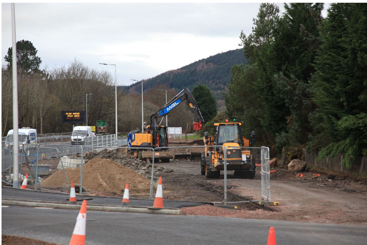
Excavation of the old A82 adjacent to the underpass
