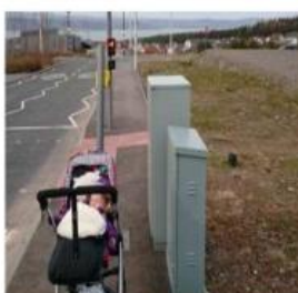
Poor infrastructure for walking/cycling
