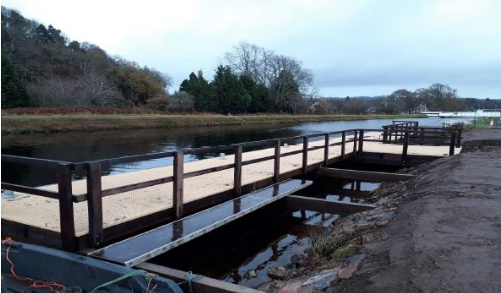
Installation of new timber jetty complete
