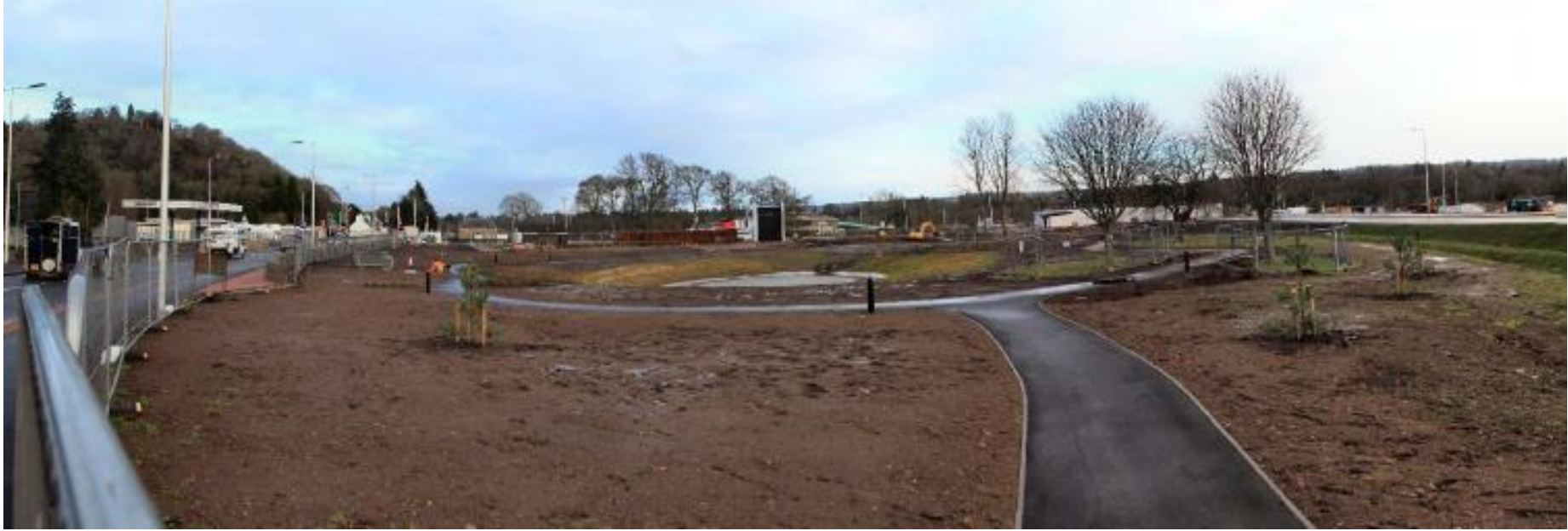
Footpaths and landscaping around ponds
