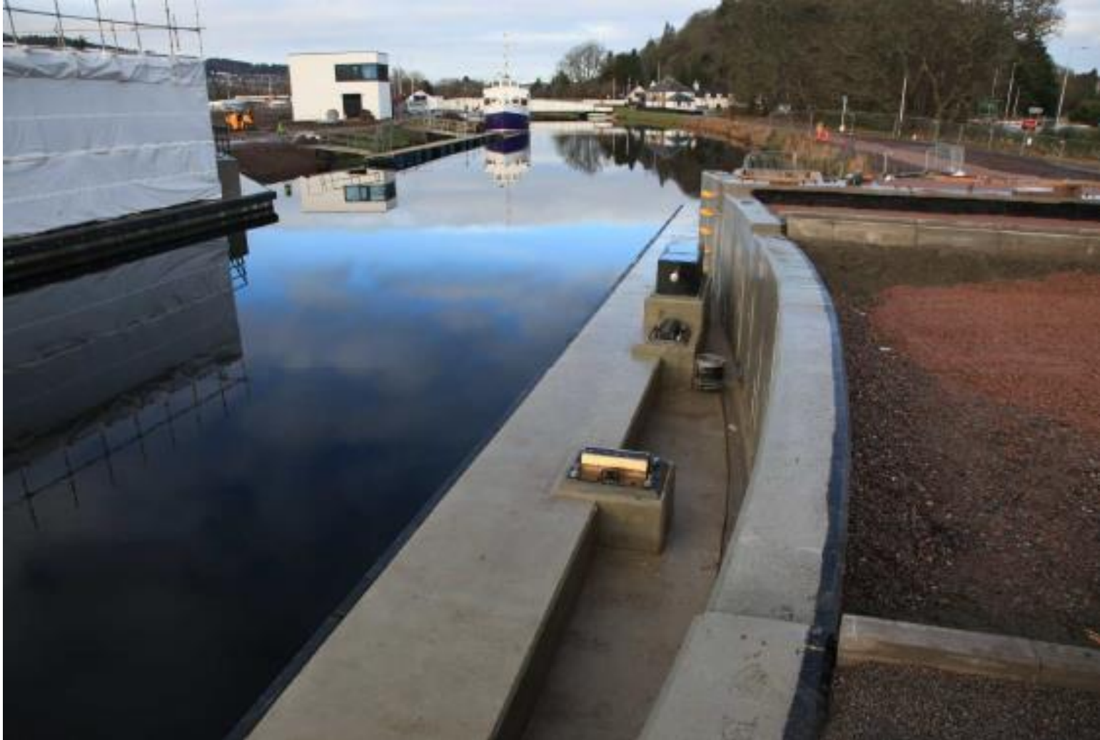
Curved East Abutment Wall with shock absorber and bearings
