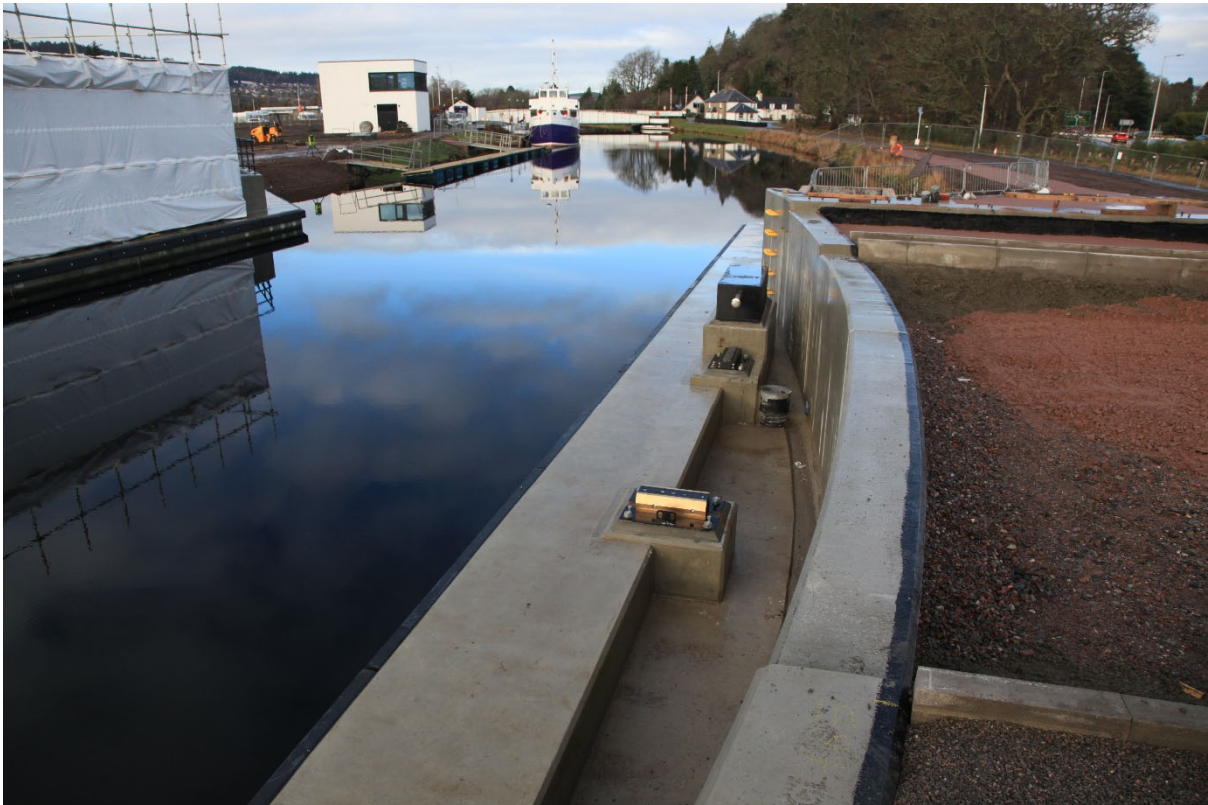
East abutment with the bearings and shock absorber clearly visible
