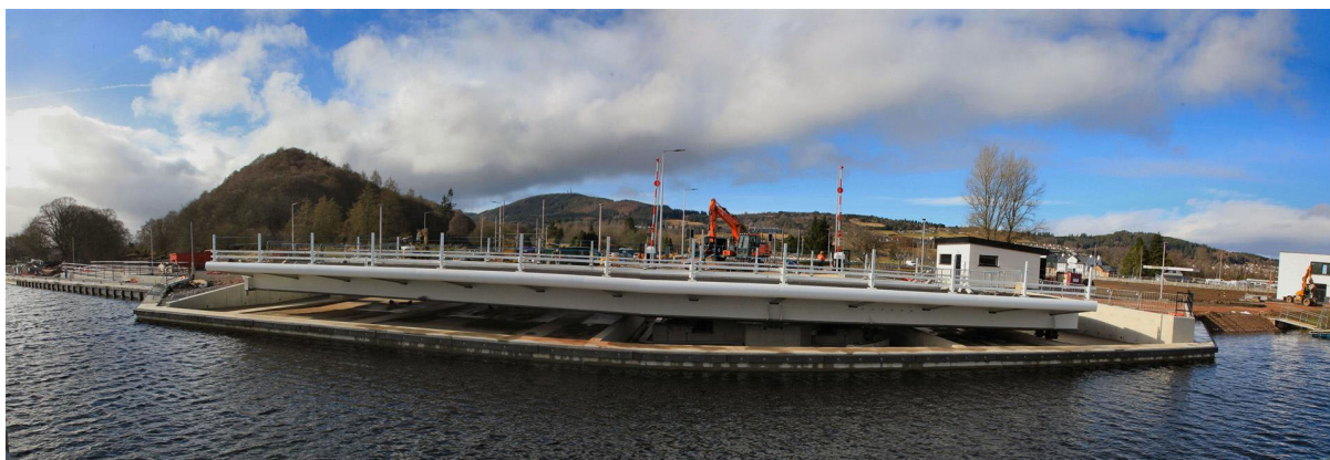
The new swing bridge sitting ready to be turned
