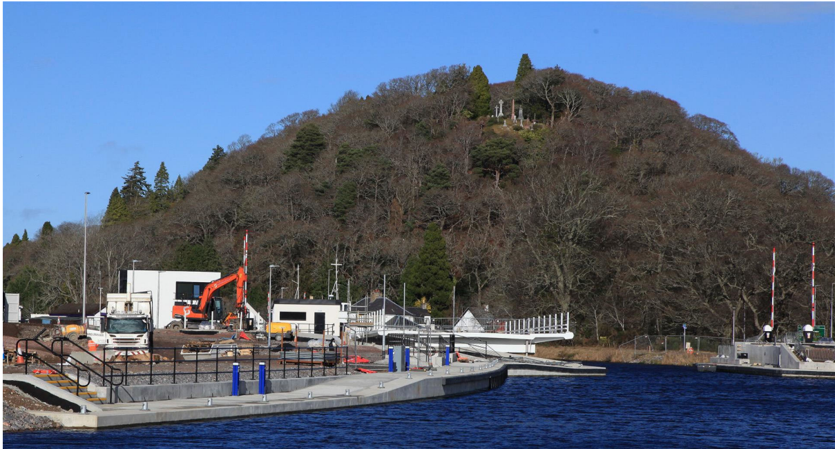
Looking North - The new wharf and nose of the bridge
