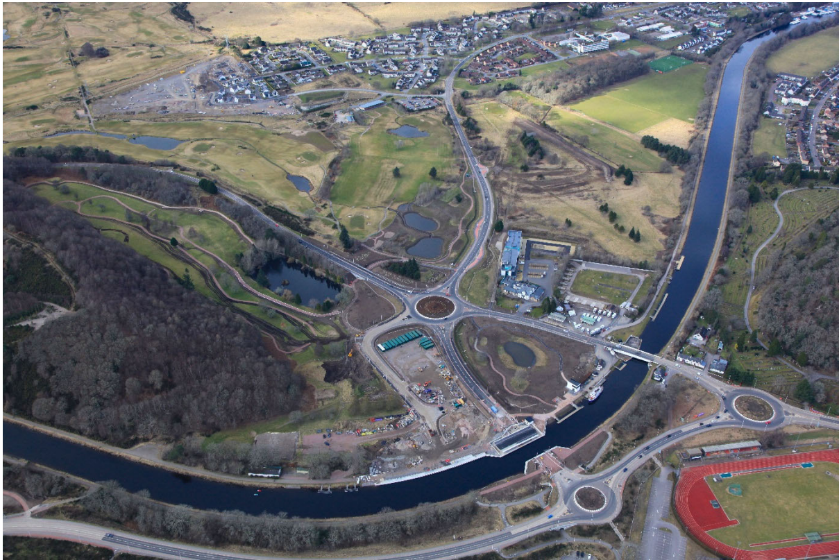
Aerial view looking West across the full site
