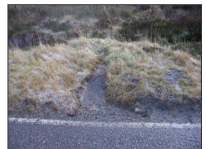
Typical Drainage Offlet
