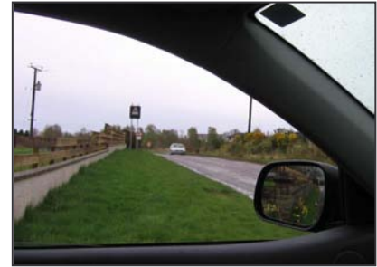
Typical Visibility Splay from the Driver's Eye view
