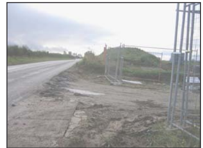
Poor site access
