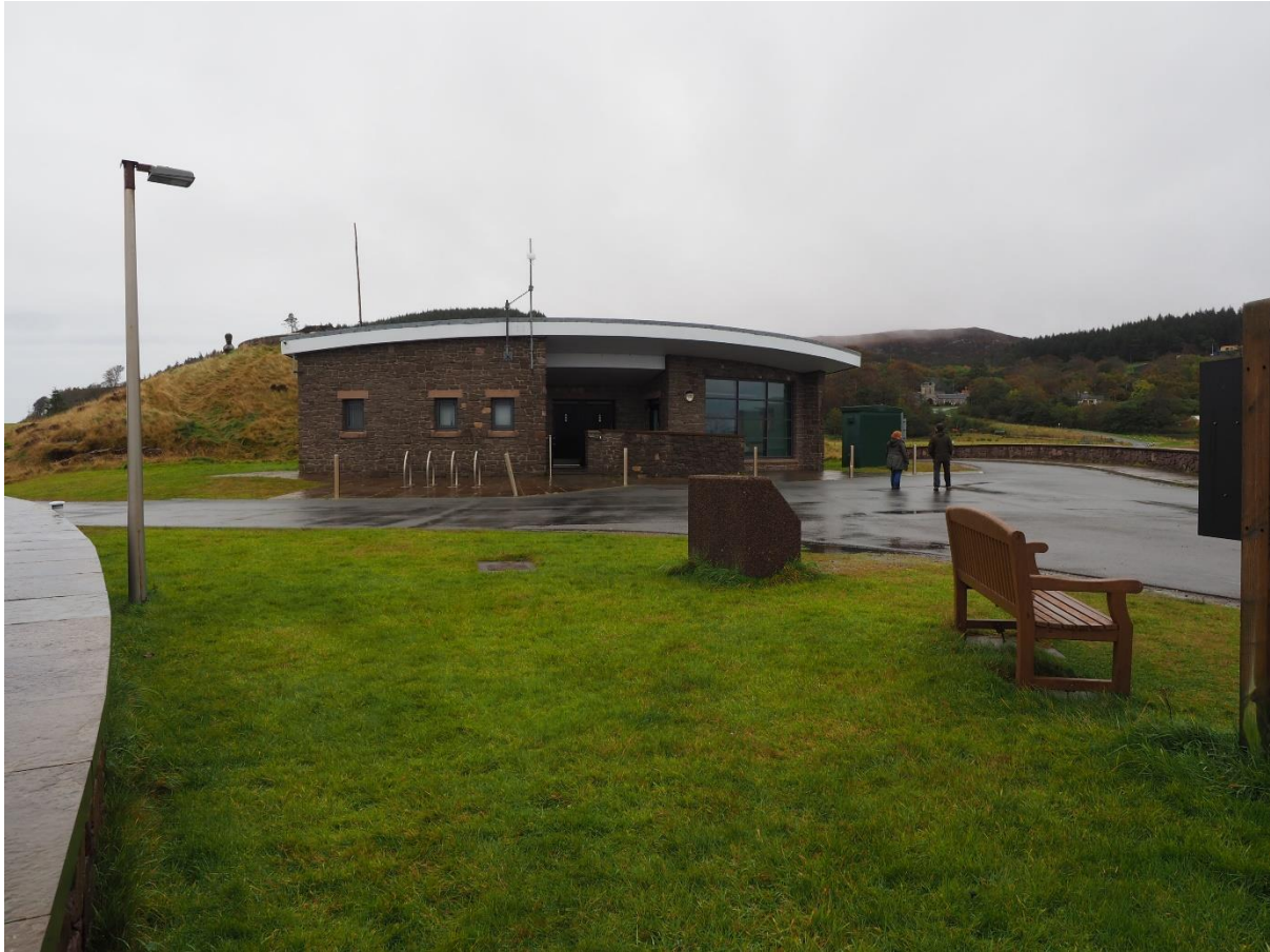
Figure 1: Raasay Ferry Terminal Building
