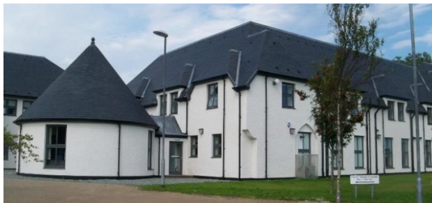
Elgin Residence (credit: Archive Centre webpage)
