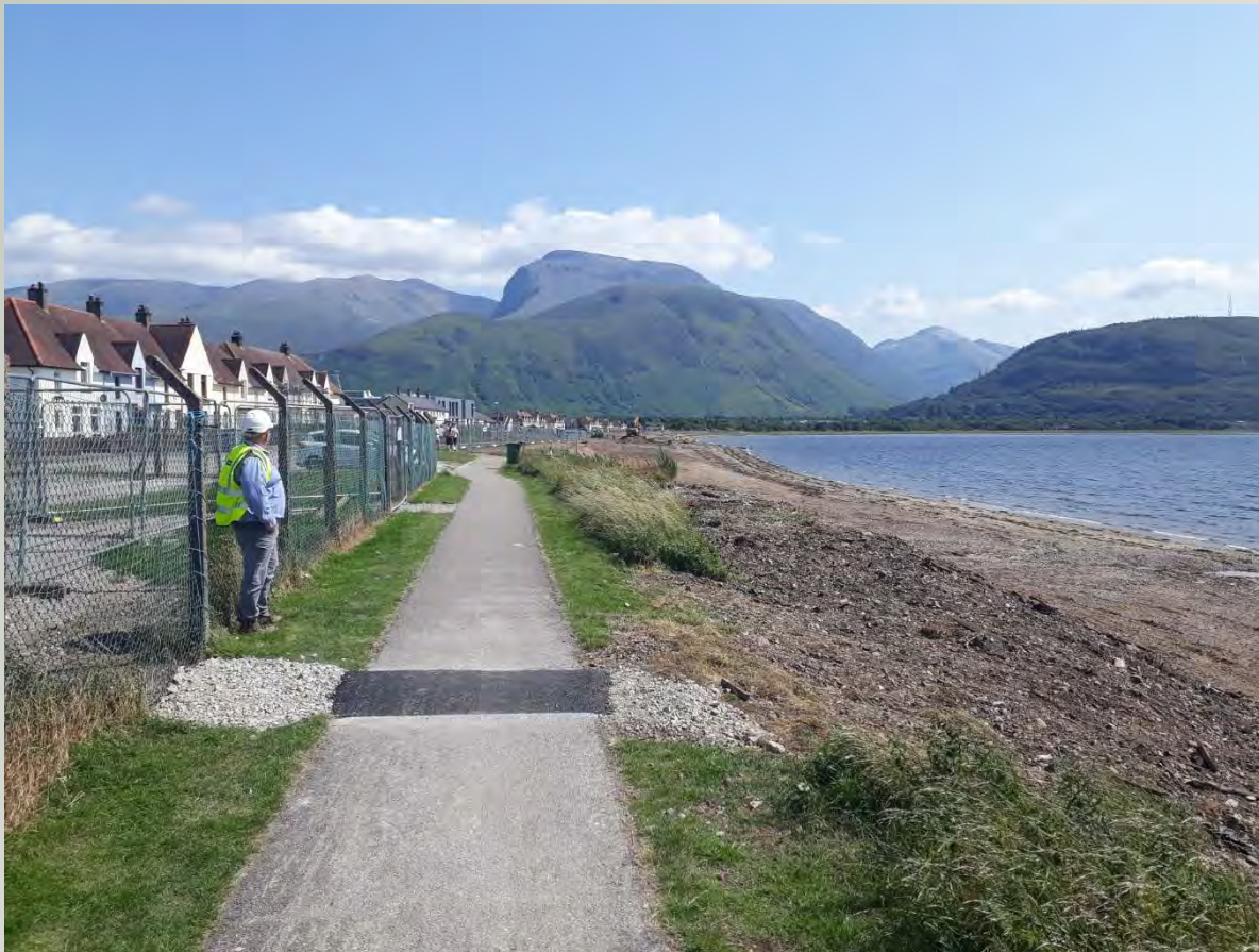
Progress Photos – Shore path reinstated following installation of sewer outfall
