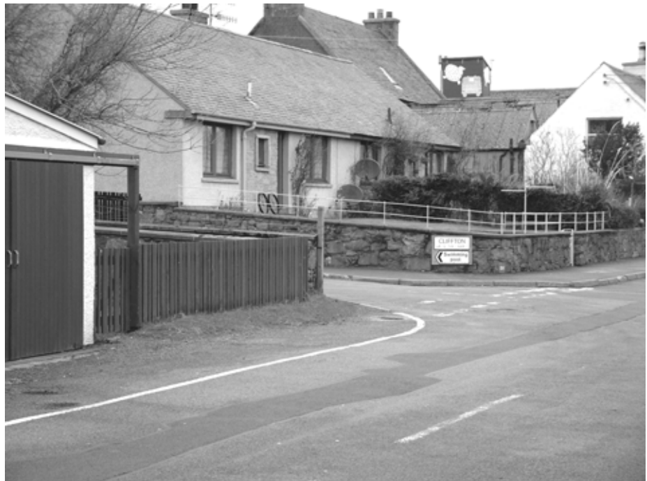
Photograph showing affected junction, where access to the Clifton area meets the main road
