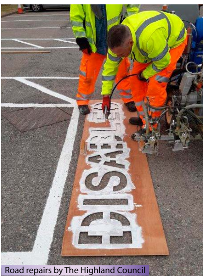
Road repairs by The Highland Council
