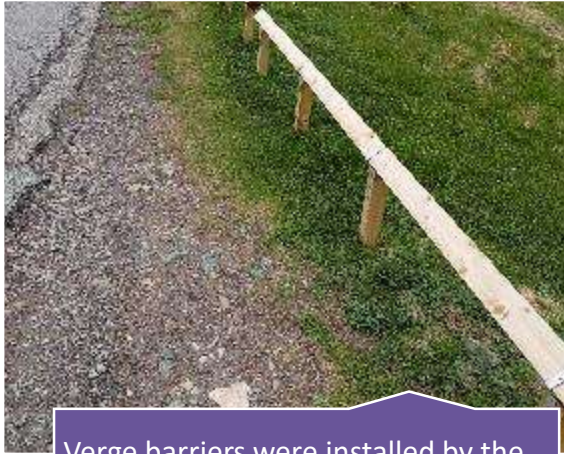
Verge barriers were installed by the community to prevent overnight parking on the machair grass.
