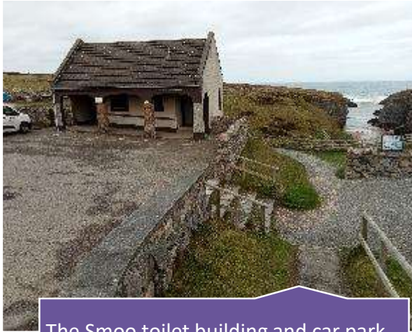
The Smoo toilet building and car park needs upgrading and carrying capacity increasing.
