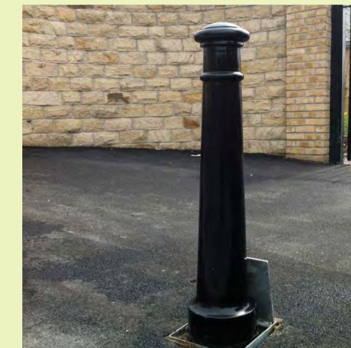
Some bollards need features such as being removable, or containing fixings to anchor other furniture to them
