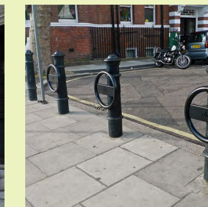
Cycle hoops can be attached to bollards for additional cycle parking
