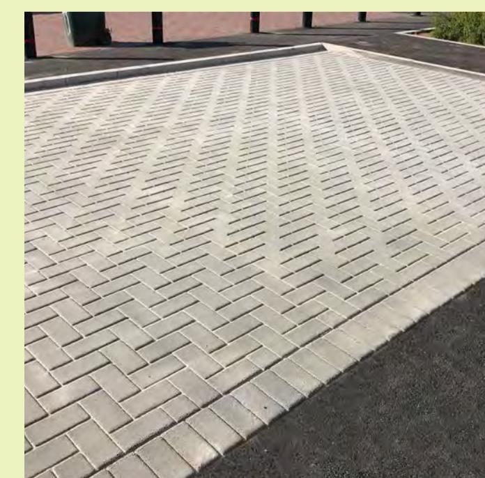
An imprinted surface in the carriageway gives the impression of paving
