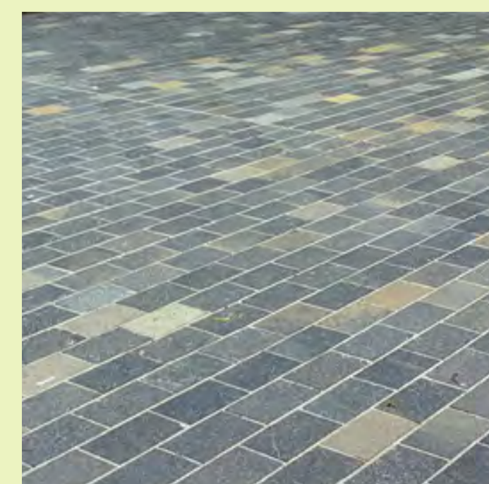
Retained existing Caithness stone should be thoroughly cleaned and repaired
