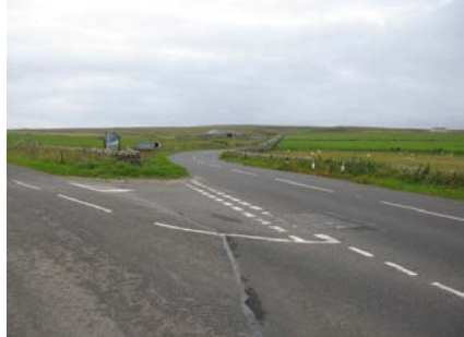
View looking west along the A836 across the junction for Janetstown
