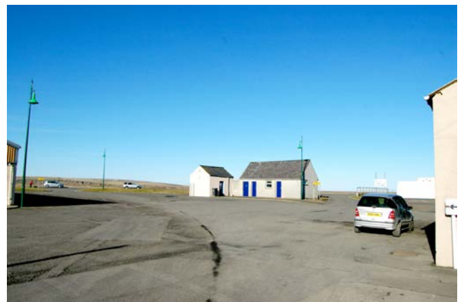
Existing buildings on promontory
