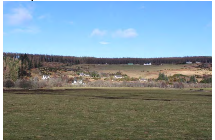
Broader floodplain pastures west of the A9 with many new residential buildings located on south-facing valley sides
