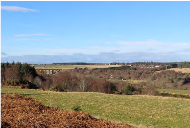
The railway swings in a broad arc through this valley - the railway viaduct crossing the River Nairn is a prominent feature.
