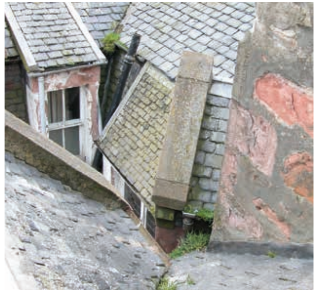
Common spaces can be difficult to inspect and create access challenges
