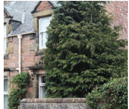
Large tree too close to house
