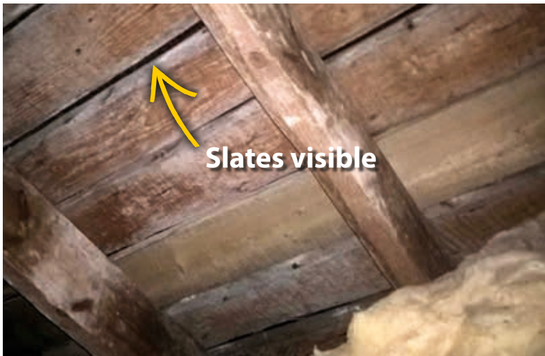
Gaps between sarking boards allow ventilation
